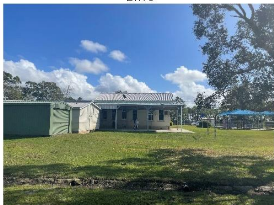
9. Rear of Building B with COLA
