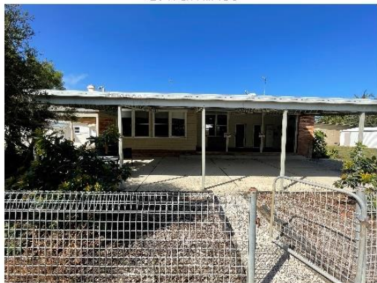
5. Entry to Building A (Classrooms) from River Drive
