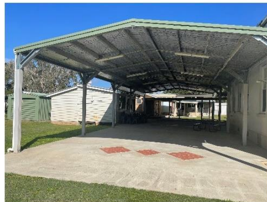
7. Covered Outdoor Learning Area (COLA) to the south of Building B
