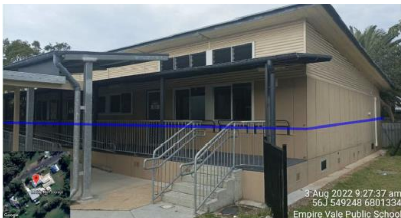
Figure 20 Building F – learning spaces with blue line indicating the approximate height of the 2022 floods with a blue line (Source: Acor Consultants)
