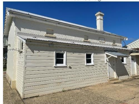
6. Building B (Library building)
