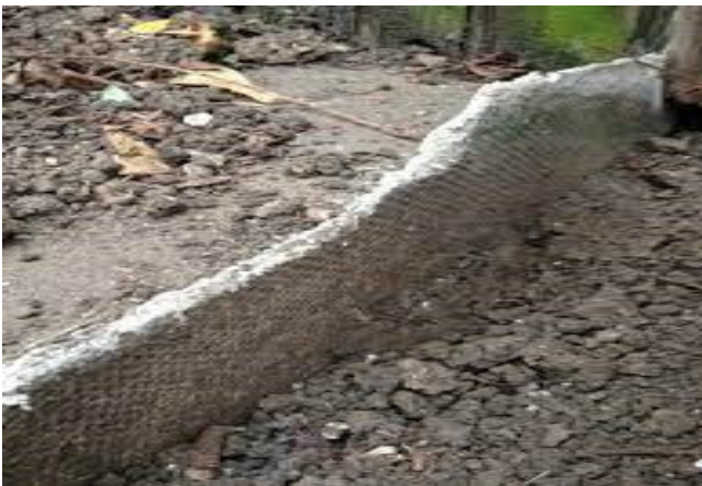
Stumps of Asbestos Cement (AC) fences , remnants of old fencing left buried in the ground.
