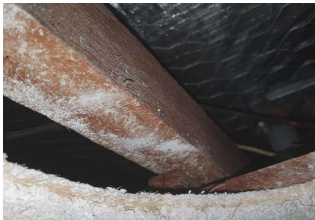
Lagging/sprayed limpet , usually found within ceiling cavities, to timber beams and to service pipes. Was used as an insulating material.
