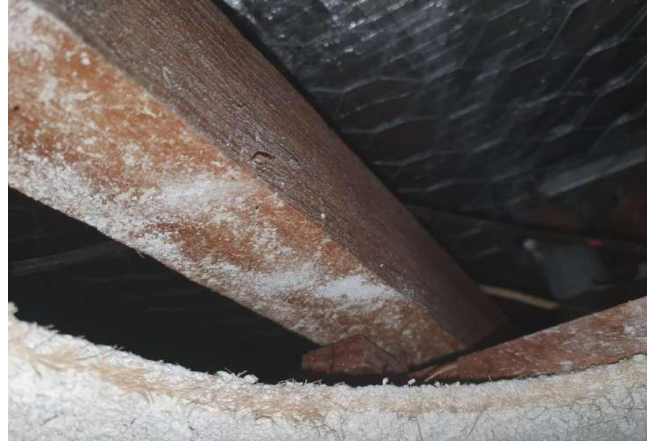
Lagging/sprayed limpet , usually found within ceiling cavities, to timber beams and to service pipes. Was used as an insulating material.
