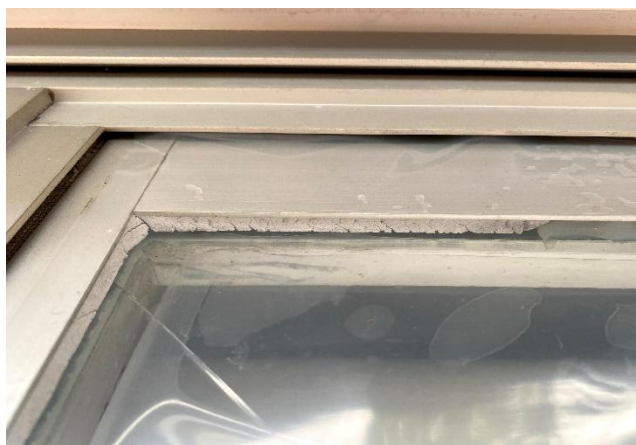
Putty , commonly used as a sealant in windows or expansion gaps.
