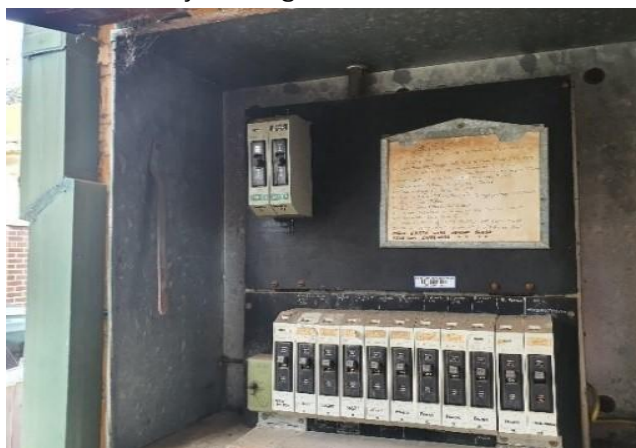
Resinous Insulation Boards , commonly used as electrical backing boards for electrical meters and circuits.
