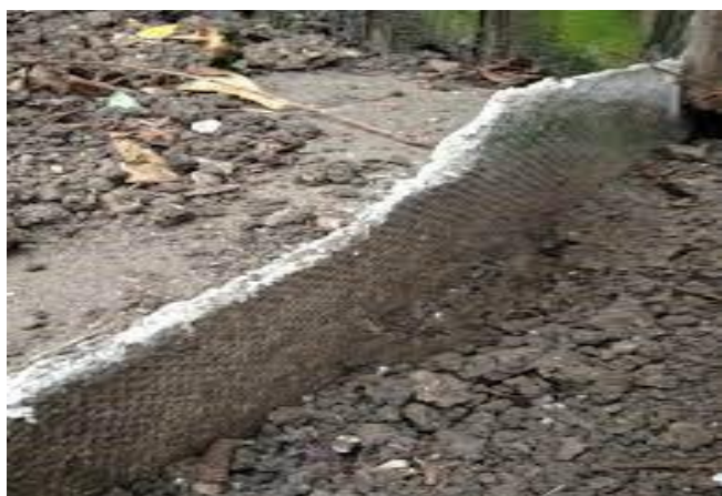
Stumps of Asbestos Cement (AC) fences , remnants of old fencing left buried in the ground.
