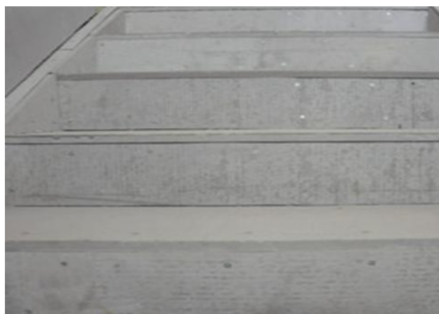
Compressed Asbestos Cement (AC) Sheet , a reinforced cement board that can be used as step treads.
