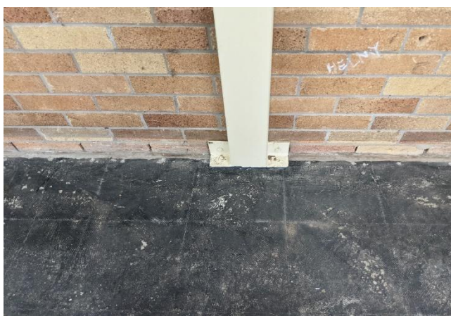
Mastic/glue , a heavy-duty adhesive commonly used to adhere vinyl floor sheeting or tiles to the substrate.
