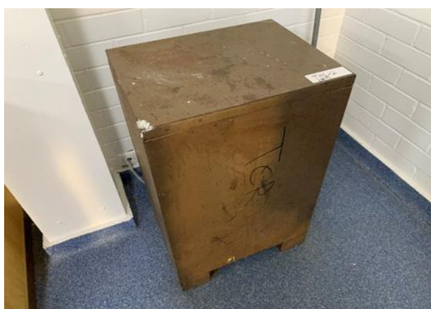
Old Electric Heaters , insulation materials in the heater may contain asbestos.
