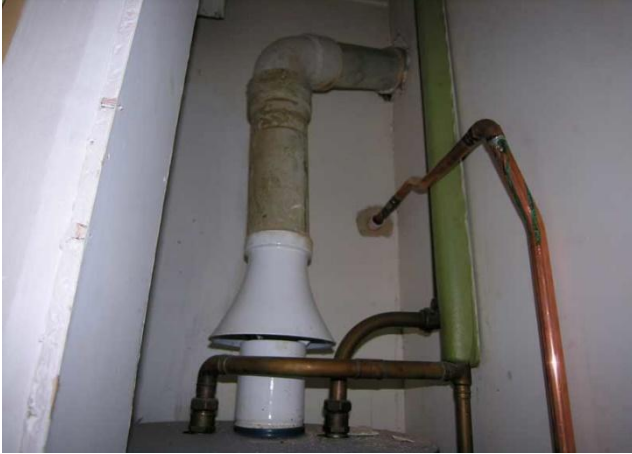
Asbestos Cement Flue , commonly used as a channel through which gases and smoke travel from a source of combustion (fireplace, fume cupboard, furnace, hot water system) to the outside environment.
