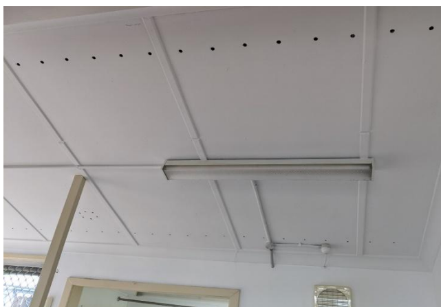
Flat Asbestos Cement (AC) Sheeting , typically used for internal and external lining of walls, eaves and ceilings.
