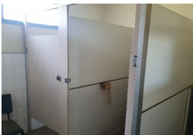
Compressed Asbestos Cement (AC) Sheet , commonly used for toilet cubicle partitions and as an underlying flooring material for walkways and classrooms with raised floors.
