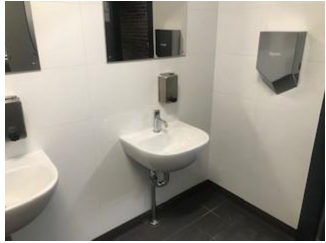
New bathroom fixtures
