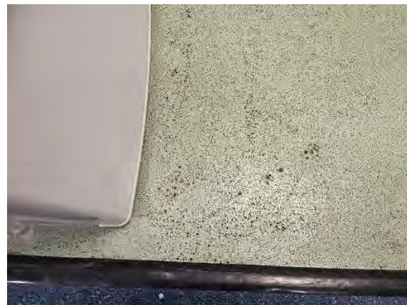
Image 29: Mould, vinyl sheet floor
