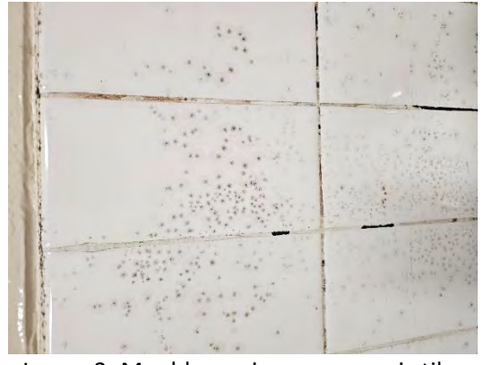
Image 2: Mould on grime on ceramic tiles
