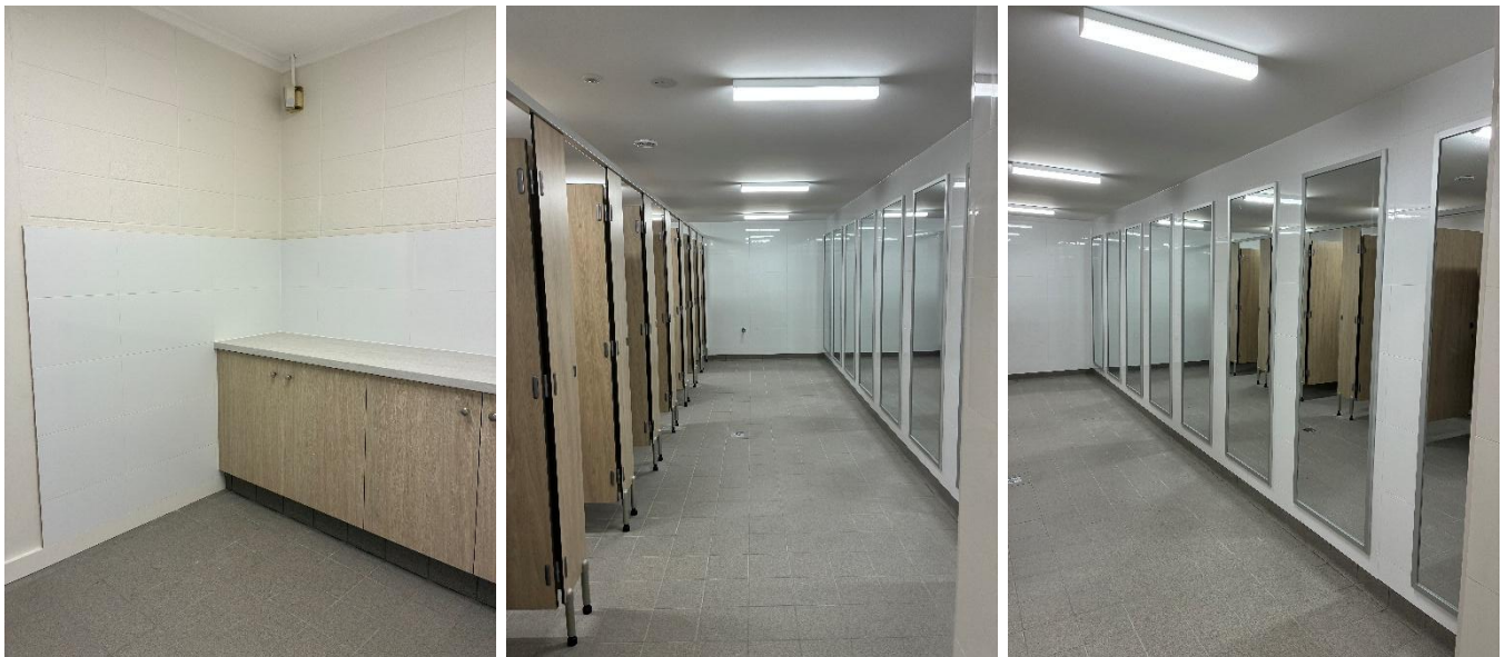
Images above: cleaner's storeroom (left) and upgraded toilets with full length mirrors (centre and right).
