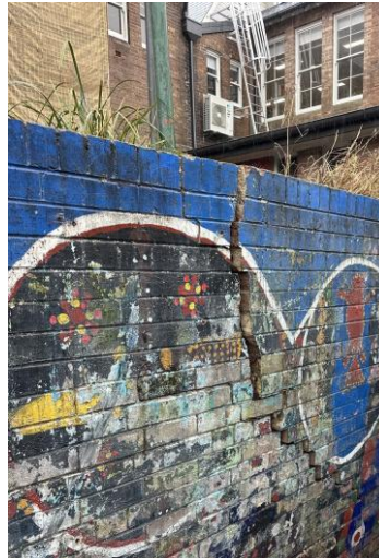
Image above: existing retaining wall which will be rebuilt.
