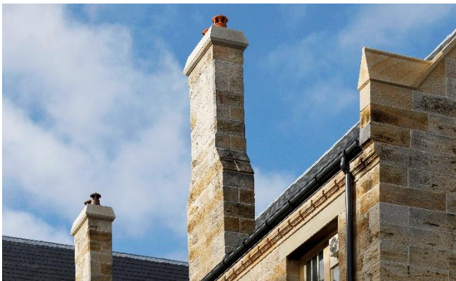
Restored chimneys on Building A
