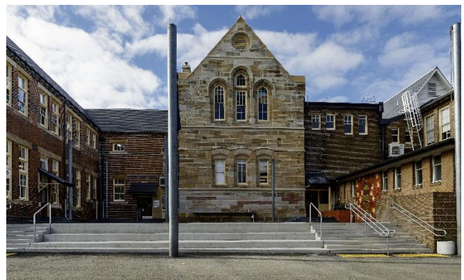
Stairs, tiered seating and improved access additions
