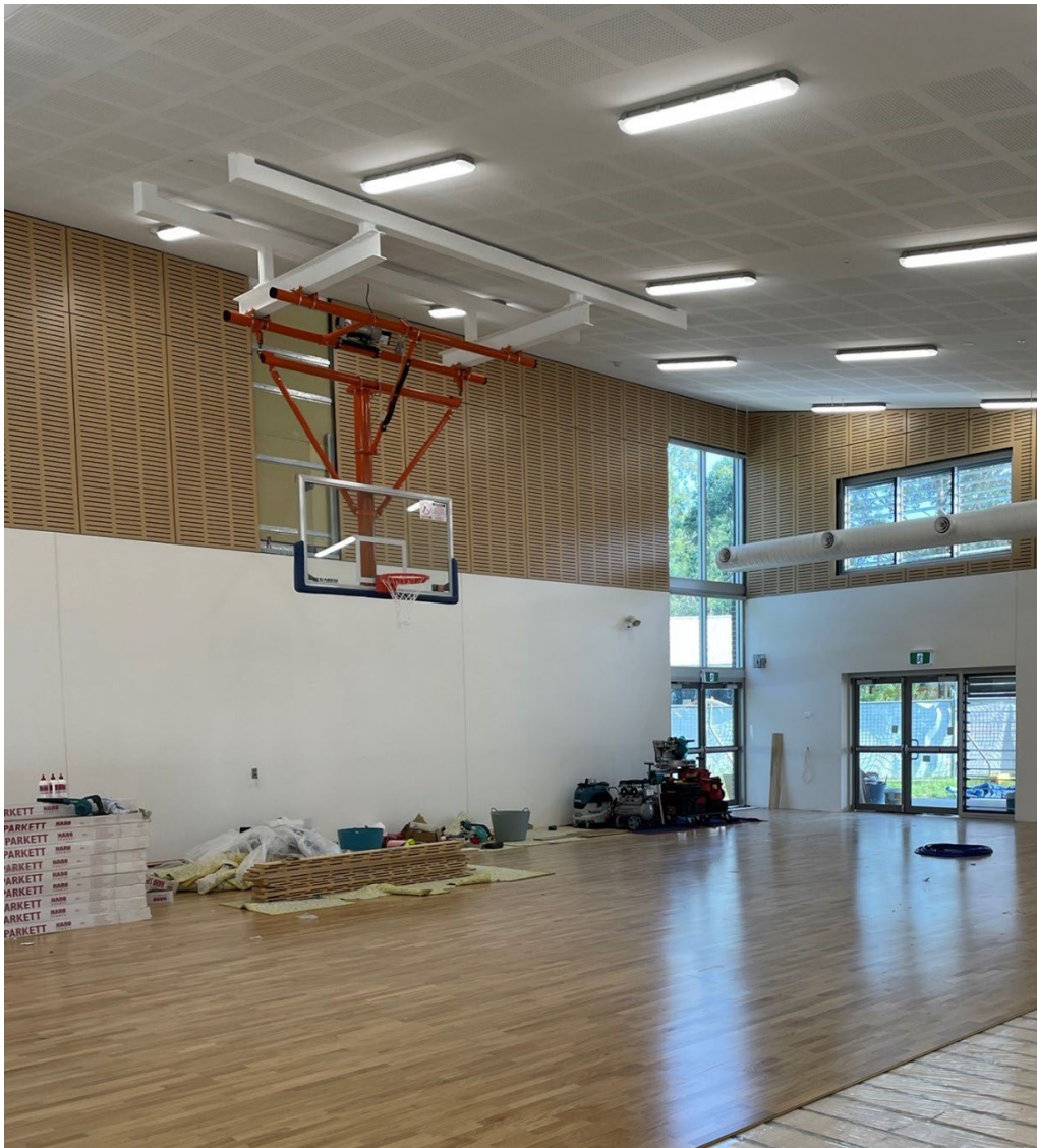
Sports floor installed
