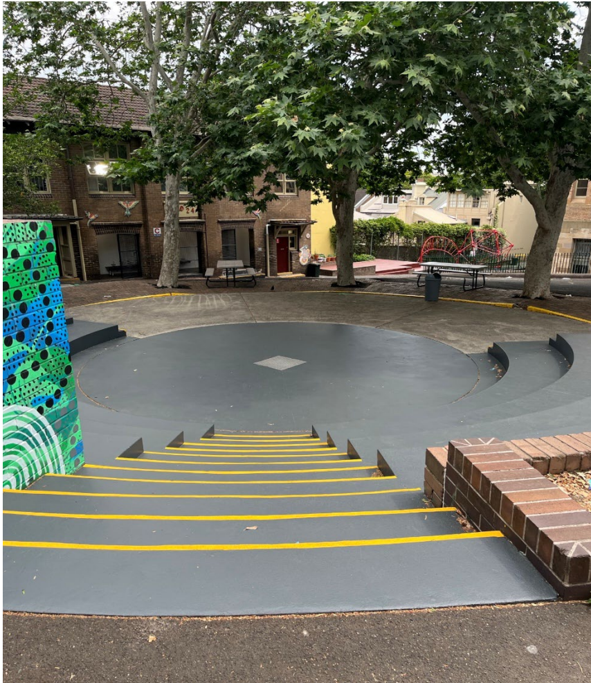
Upgrades to the tiered seating and safety strips done over the school holidays
