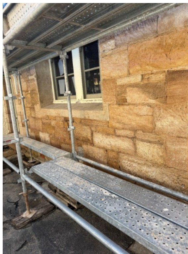
Masonry paint removal
