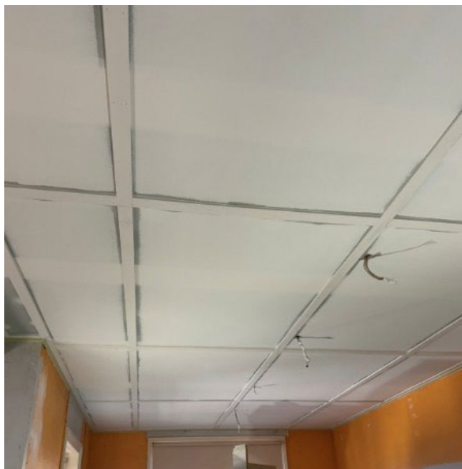
New ceiling installation
