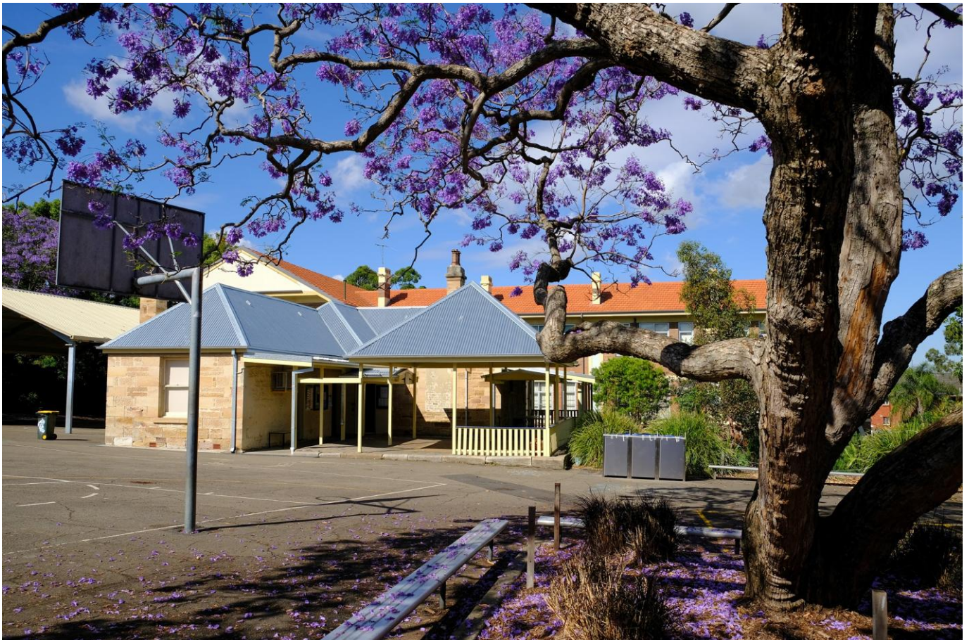
Building B at Gladesville Public School, also known as the OOSH Building
