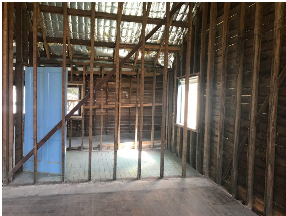
Above: the administration building stripped out and cleaned
