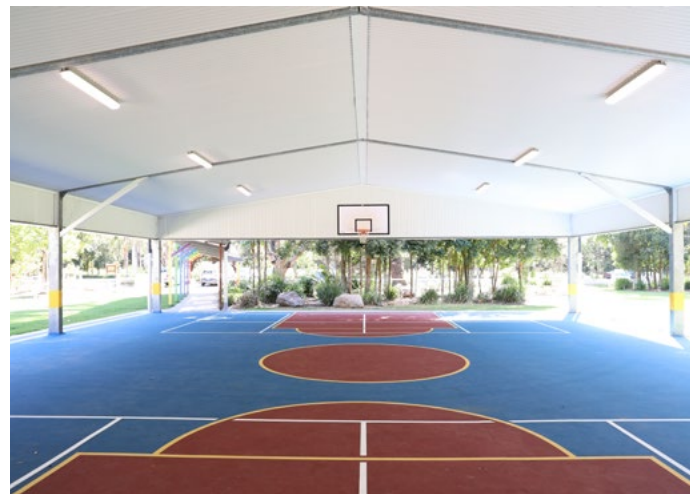
Resurfaced sports court and acoustic lined COLA
