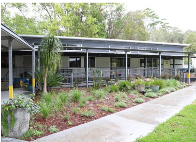
Remediated administration building and classroom
