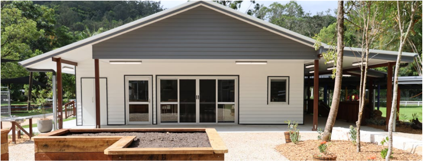
Rebuilt Classroom Block A
