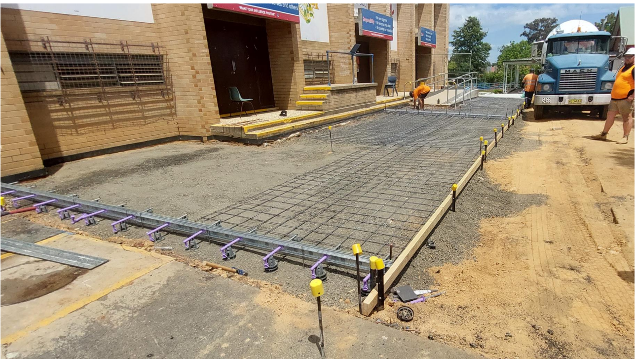
Photo 7: Pavement works to the access way of Block EE underway.
