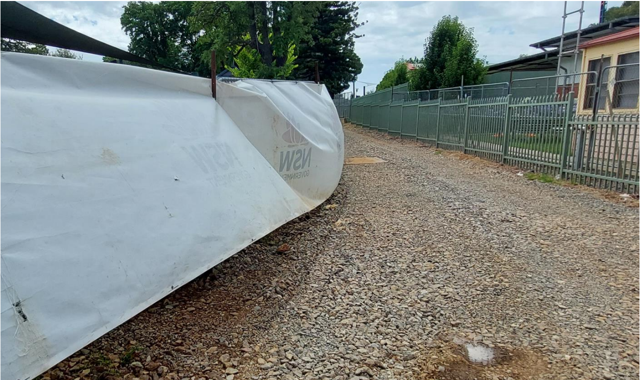
Photo 1: Shadecloth and stabilised haul road. Note childcare centre to right of shot and absence of hoarding / barriers.
