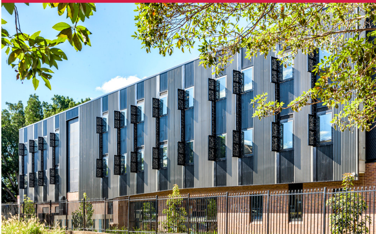
West Ryde Public School upgrade
