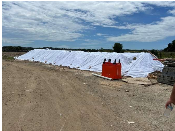
Photo 9: A stockpile of Excavated Natural Material (ENM) was covered in geofabric to reduce potential for erosion and dust.
