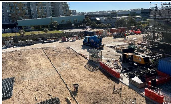
Photos 2 and 3: The western side (active side) of the site, commencing from the main driveway, was being progressively sealed with concrete to minimise tracking and dust. RobertsCo advised they proposed to seal the entire western side. Formwork was observed where additional concrete was scheduled to be laid later in the day.
