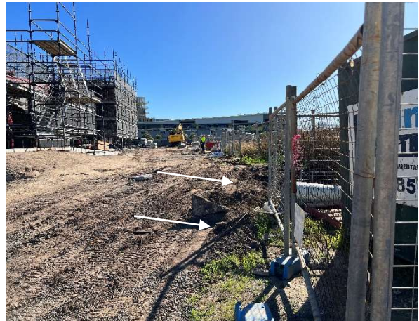
Photo 12: Northern boundary (eastern end) – In the northeastern corner of the site, the site grades towards the neighbouring property and there is potential for sediment laden runoff to leave the site.
