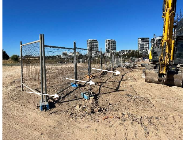
Photo 11: Northern boundary (western end) – Stormwater runoff from the neighbouring property can enter the site potentially increasing hydraulic load on the site's erosion and sediment controls.
