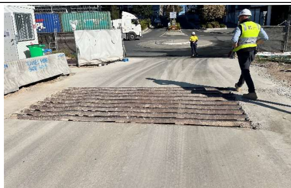
Photos 2 and 3: The western side (active side) of the site, commencing from the main driveway, was being progressively sealed with concrete to minimise tracking and dust. RobertsCo advised they proposed to seal the entire western side. Formwork was observed where additional concrete was scheduled to be laid later in the day.
