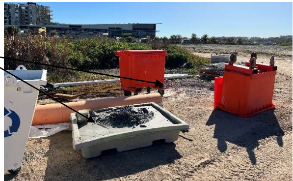
Photo 14: A small quantity of concrete waste (agitator wash-out) was observed on the adjacent property within a plastic bin. A small quantity was also dumped on the ground.
