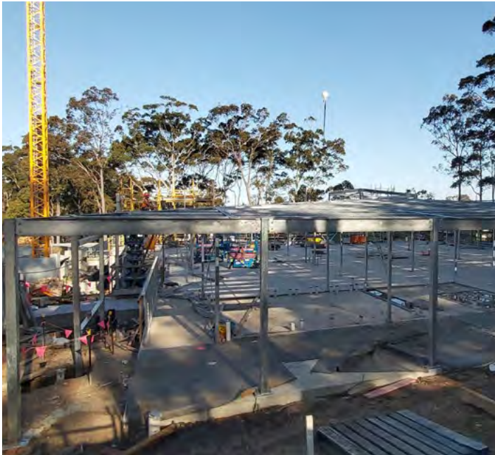
Steel framework for roof of new Block K
