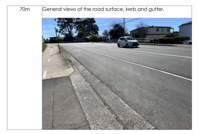
Views of the layback and gutter showing multiple cracks.
