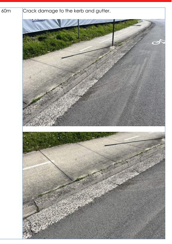
60m Crack damage to the kerb and gutter.
