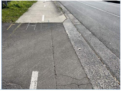
Views of the driveway crossover showing crack damage and potholes throughout.
