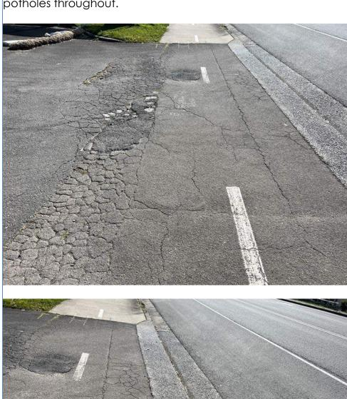
Views of the driveway crossover showing crack damage and potholes throughout.
