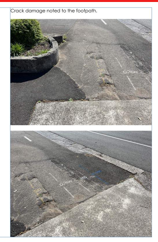
30m Views of the driveway crossover showing crack damage and potholes throughout.
