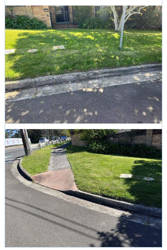
Crack damage throughout the kerb and gutter to the north side of Arnhem Road, Allambie Heights.
