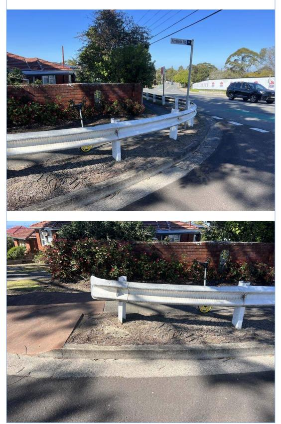
Kerb and gutter showing crack damage and lifting of the expansion joints of Arnhem Road, south side.
