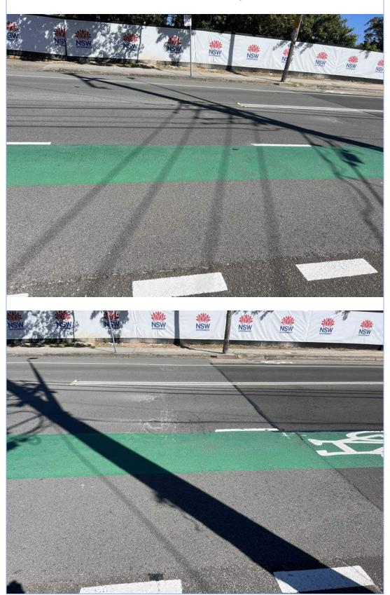
Crocodile cracking and subsidence to the road surface at the intersection of Arnhem Road and Allambie Road, Allambie Heights.
