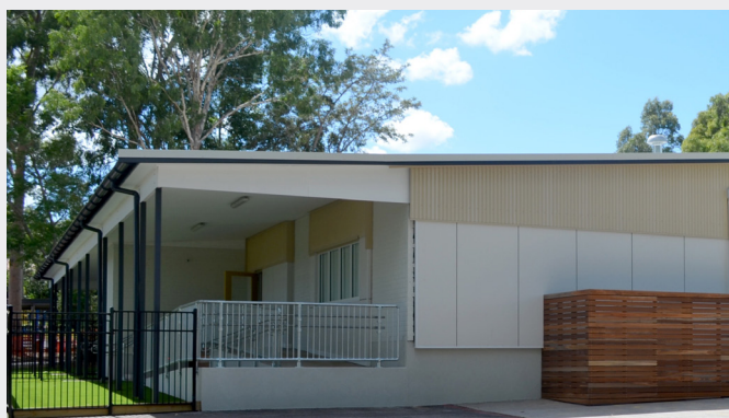
Recently completed special education facilities and play area
