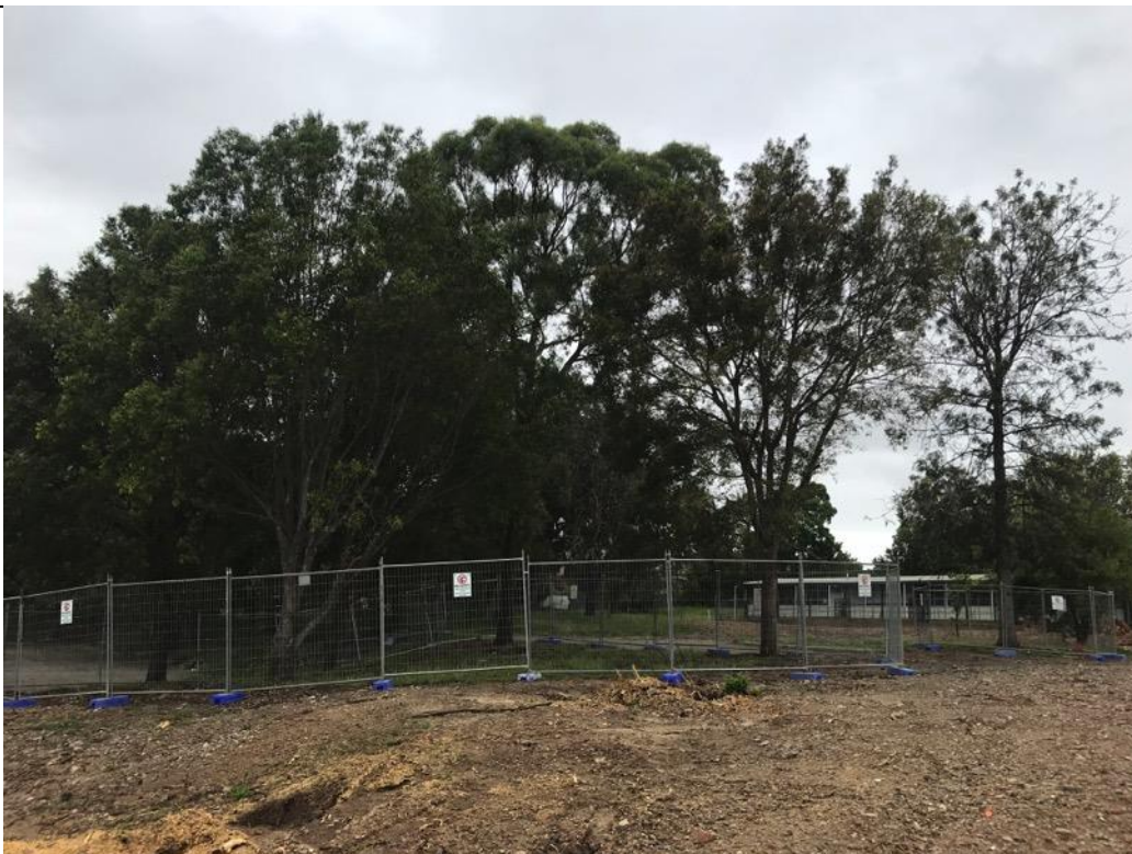
Image L: Tree protection fencing installed adjacent to tree 70, 70A, 71, 72, 73, 75 and 198.
