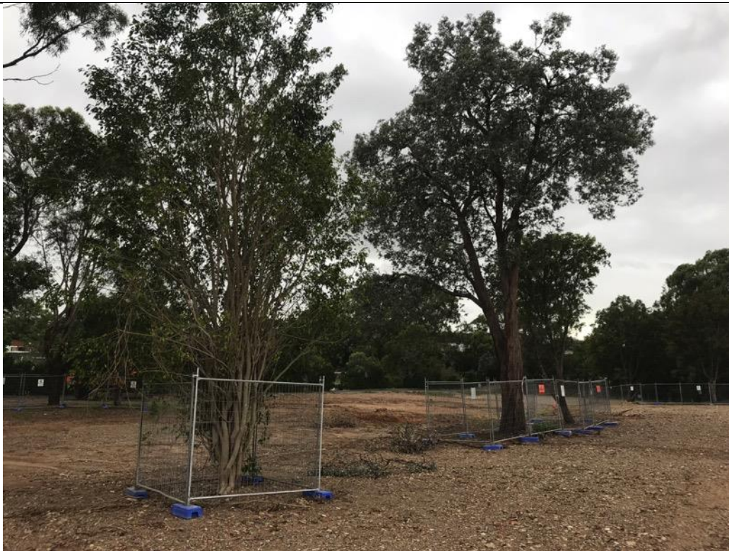
Image K: Tree protection fencing installed adjacent to tree 120, 141 and 142.
