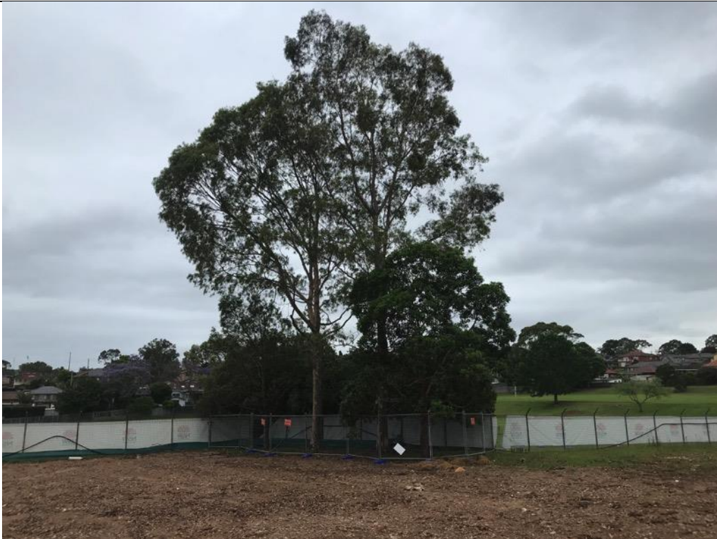
Image G: Tree protection fencing installed adjacent to tree 94, 95, 96 and 121A.
