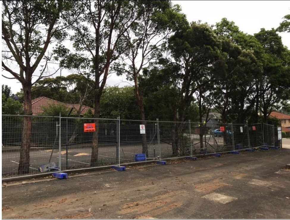
Image A: Tree protection fencing installed adjacent to tree 145 - 153.
