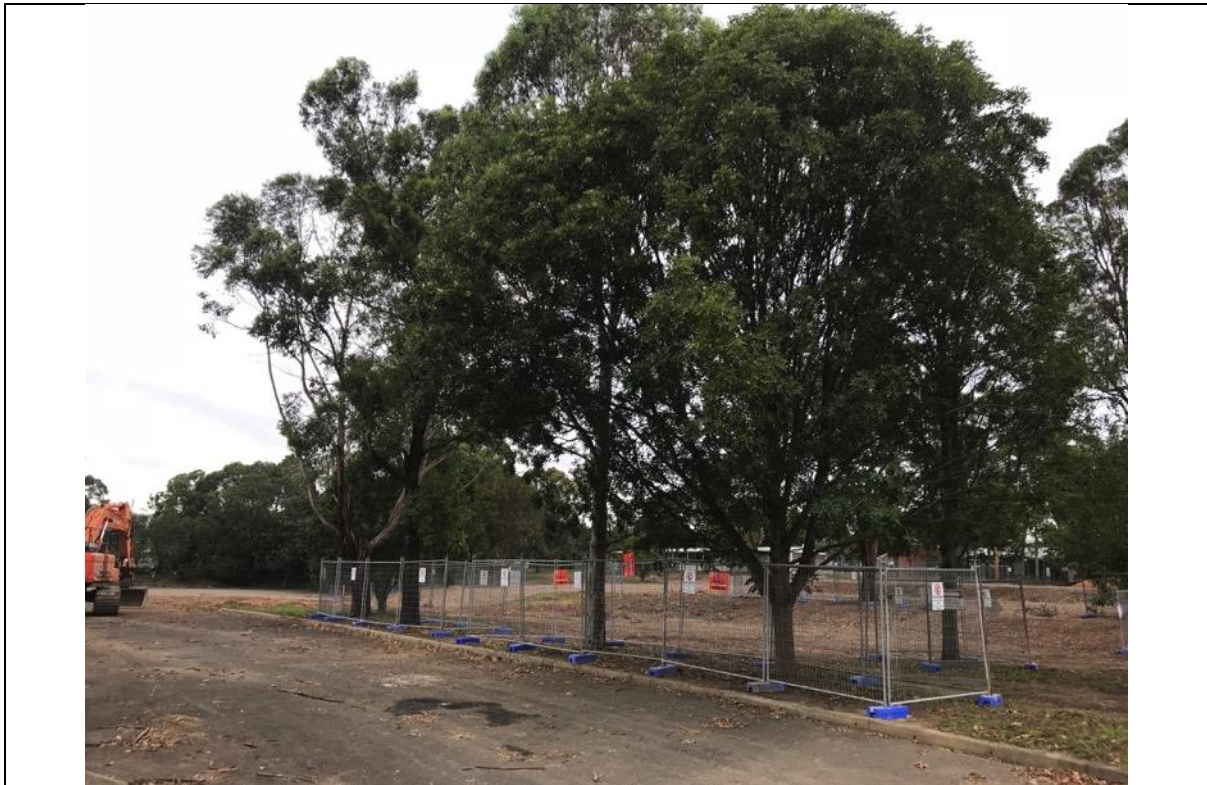
Image I: Tree protection fencing installed adjacent to tree 108, 109, 110, 111, 111A and 119.
