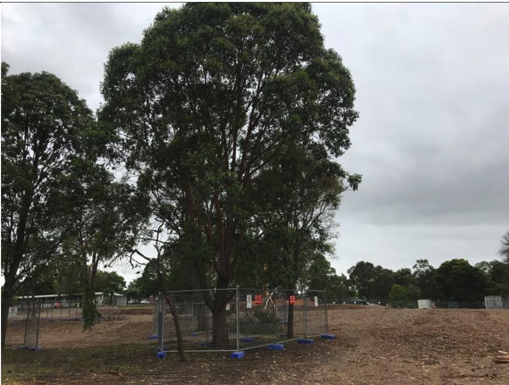
Image H: Tree protection fencing installed adjacent to tree 115 and 116.
