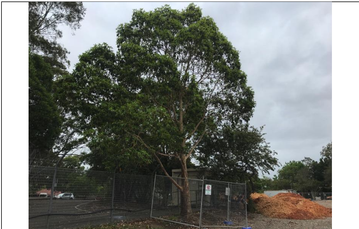
Image M: Tree protection fencing installed adjacent to tree 182.
