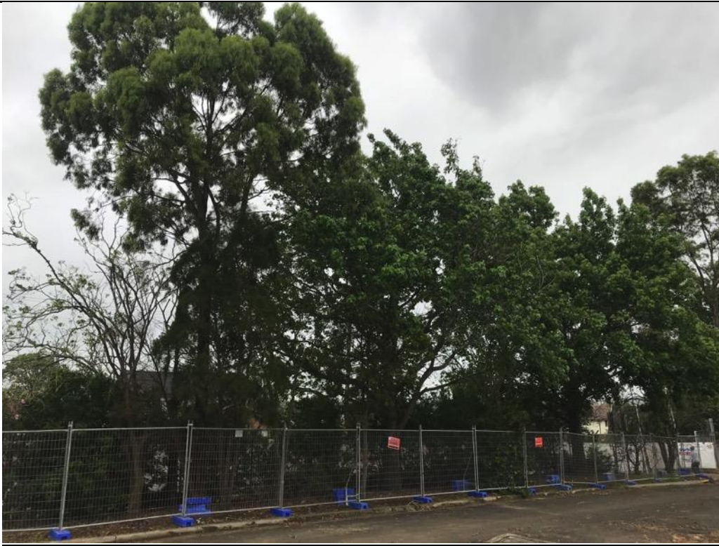
Image E: Tree protection fencing installed adjacent to tree 101, 102, 133, 134 and 134A.
