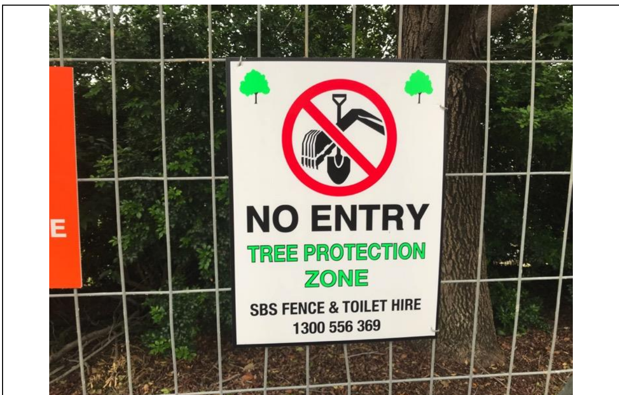
Image N: TPZ signage used on site.
