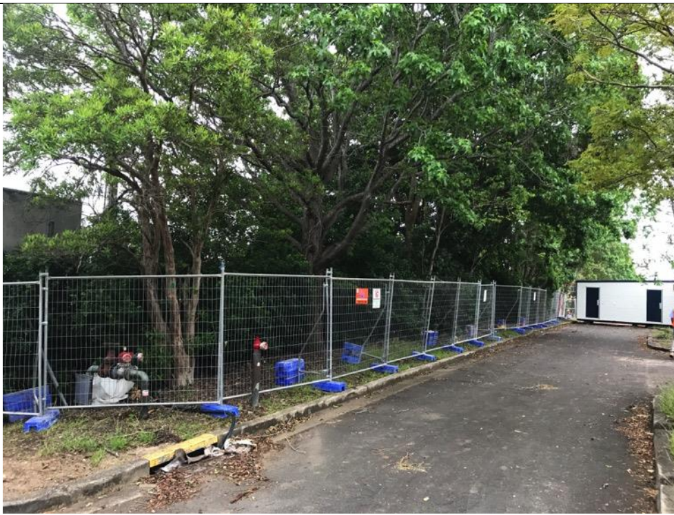
Image B: Tree protection fencing installed adjacent to tree 158, 159, 160, 161, 162, 169, 170, 171 and 172.
