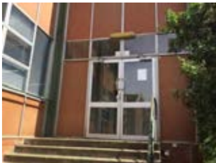
PHOTO NO.: J154351-001-PHOTO130 RESULT: ASBESTOS - POSITIVE BUILDING/LEVEL: B00B - ALL LEVELS ROOM/LOCATION: ALL AREAS - VARIOUS THROUGHOUT FEATURE/MATERIAL: INFILL PANELS - COMPRESSED CEMENT SHEETING SAMPLE NO.: PREVIOUSLY SAMPLED GREENCAP J146932-02-002-024
