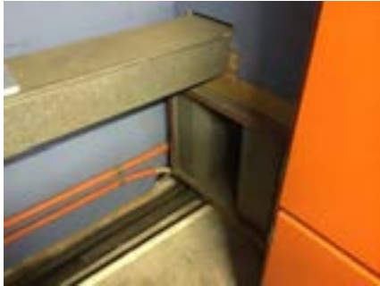
PHOTO NO.: J154351-001-PHOTO180 RESULT: SMF - POSITIVE BUILDING/LEVEL: B00D - GROUND LEVEL ROOM/LOCATION: DR0023 - PLANT ROOM - NORTH FEATURE/MATERIAL: DUCTWORK INSULATION - INSULATION MATERIAL SAMPLE NO.: -
