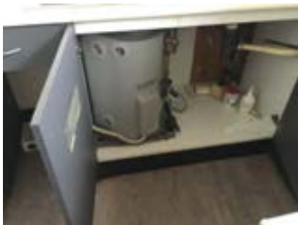
PHOTO NO.: J154351-001-PHOTO106 RESULT: SMF - PRESUMED POSITIVE BUILDING/LEVEL: B00B - LEVEL ONE ROOM/LOCATION: BR1020 - KITCHEN - BELOW SINK FEATURE/MATERIAL: HOT WATER SERVICE INSULATION - INSULATION MATERIAL SAMPLE NO.: -
