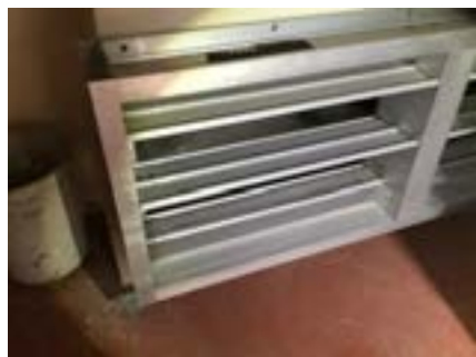
PHOTO NO.: J154351-001-PHOTO073 RESULT: SMF - POSITIVE BUILDING/LEVEL: B00E - GROUND LEVEL ROOM/LOCATION: ER0002 - PLANT ROOM - VARIOUS THROUGHOUT FEATURE/MATERIAL: DUCTWORK INSULATION - INSULATION MATERIAL SAMPLE NO.: -
