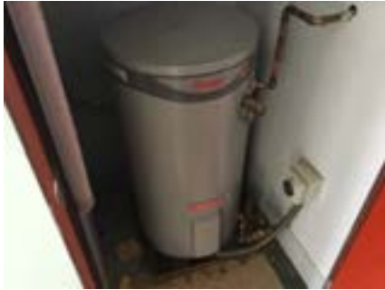
PHOTO NO.: J154351-001-PHOTO007 RESULT: SMF - PRESUMED POSITIVE BUILDING/LEVEL: B00K - GROUND LEVEL ROOM/LOCATION: KR0007 - SERVICE AREA - CENTRAL FEATURE/MATERIAL: HOT WATER SERVICE INSULATION - INSULATION MATERIAL SAMPLE NO.: -
