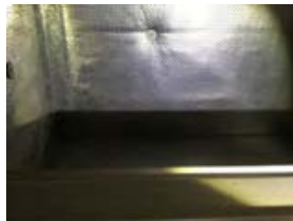
PHOTO NO.: J154351-001-PHOTO072 RESULT: SMF - POSITIVE BUILDING/LEVEL: B00E - GROUND LEVEL ROOM/LOCATION: ER0002 - PLANT ROOM - VARIOUS THROUGHOUT FEATURE/MATERIAL: DUCTWORK INSULATION - INSULATION MATERIAL SAMPLE NO.: -
