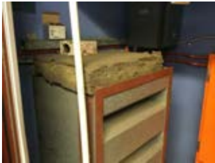
PHOTO NO.: J154351-001-PHOTO166 RESULT: SMF - POSITIVE BUILDING/LEVEL: B00D - GROUND LEVEL ROOM/LOCATION: DR0017 - PLANT ROOM - VARIOUS THROUGHOUT FEATURE/MATERIAL: INSULATION - INSULATION MATERIAL SAMPLE NO.: -
