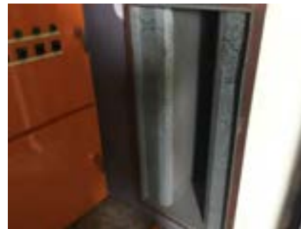
PHOTO NO.: J154351-001-PHOTO087 RESULT: SMF - POSITIVE BUILDING/LEVEL: B00E - LEVEL ONE ROOM/LOCATION: ER1004 - PLANT ROOM - VARIOUS THROUGHOUT FEATURE/MATERIAL: DUCTWORK INSULATION - INSULATION MATERIAL SAMPLE NO.: -
