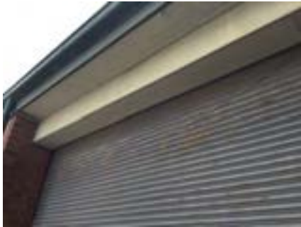
PHOTO NO.: J154351-001-PHOTO187 RESULT: ASBESTOS - PRESUMED POSITIVE BUILDING/LEVEL: B00D - LEVEL ONE ROOM/LOCATION: ALL AREAS - VARIOUS THROUGHOUT FEATURE/MATERIAL: EAVES - FIBRE CEMENT SHEETING SAMPLE NO.: NOT SAMPLED HEIGHT RESTRICTED
