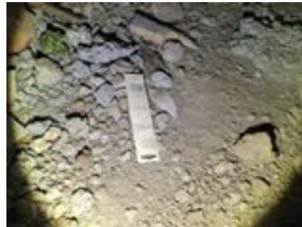
PHOTO NO.: J154351-001-PHOTO051 RESULT: ASBESTOS - POSITIVE BUILDING/LEVEL: B00A - SUB-FLOOR ROOM/LOCATION: ALL AREAS - VARIOUS THROUGHOUT FEATURE/MATERIAL: DEBRIS - FIBRE CEMENT SHEETING SAMPLE NO.: J154351-001-017
