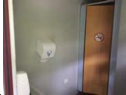
PHOTO NO.: J154351-001-PHOTO006 RESULT: SMF - POSITIVE BUILDING/LEVEL: B00K - GROUND LEVEL ROOM/LOCATION: KR0008 - MENS LOCKER/AIRLOCK AREA - VARIOUS THROUGHOUT FEATURE/MATERIAL: INSULATION - INSULATION MATERIAL SAMPLE NO.: -
