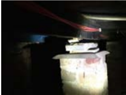
PHOTO NO.: J154351-001-PHOTO047 RESULT: ASBESTOS - POSITIVE BUILDING/LEVEL: B00A - SUB-FLOOR ROOM/LOCATION: ALL AREAS - VARIOUS THROUGHOUT FEATURE/MATERIAL: PACKER - FIBRE CEMENT SHEETING SAMPLE NO.: J154351-001-014
