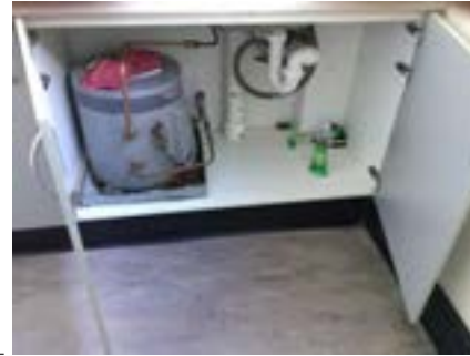
PHOTO NO.: J154351-001-PHOTO155 RESULT: SMF - PRESUMED POSITIVE BUILDING/LEVEL: B00D - LEVEL ONE ROOM/LOCATION: DR1002 - KITCHEN - BELOW SINK FEATURE/MATERIAL: HOT WATER SERVICE INSULATION - INSULATION MATERIAL SAMPLE NO.: -
