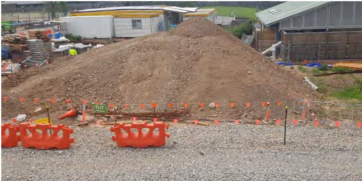
Photo 7: Unstabilised stockpile
