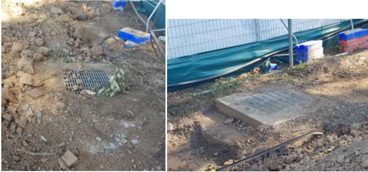
Photo 10: Series showing examples of ERSED controls requiring improvement.
