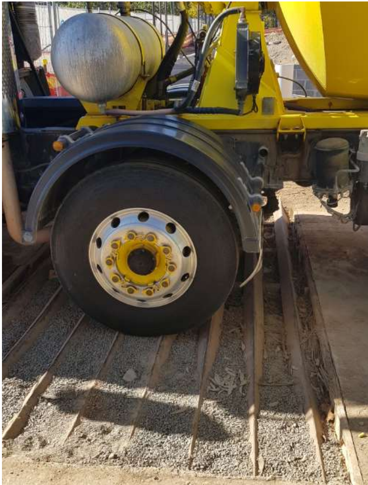
Photo 8: Rumble grid requiring maintenance and assessment against CSWMSP.
