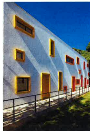
AW2 COLOURED CLADDING OVER FRAME
