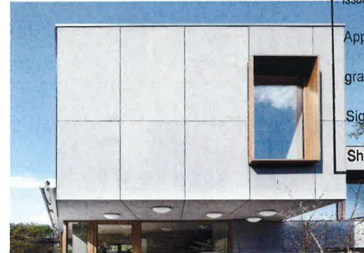
FC PREFINISHED FIBRE CEMENT SHEET
