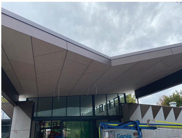
A sneak peek of the new STEM building under construction.
