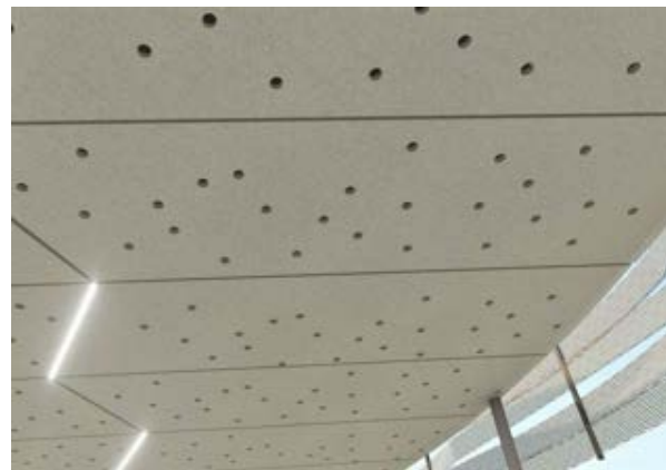
PERFORATED FC SOFFIT, FACTORY PAINTED
