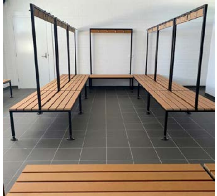
Completed fitness learning hub and changerooms
