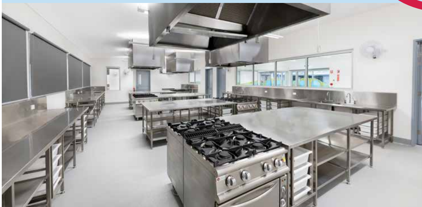
An example of food technology facilities delivered at NSW schools
