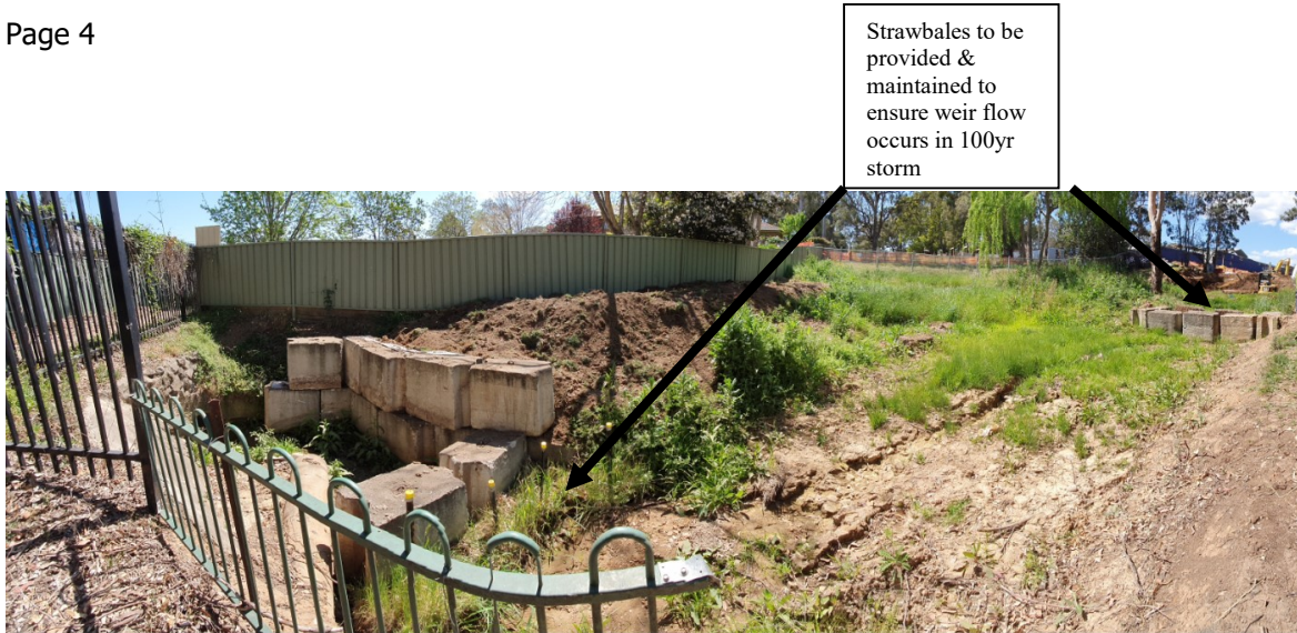
Figure 3 Overland flow channel
