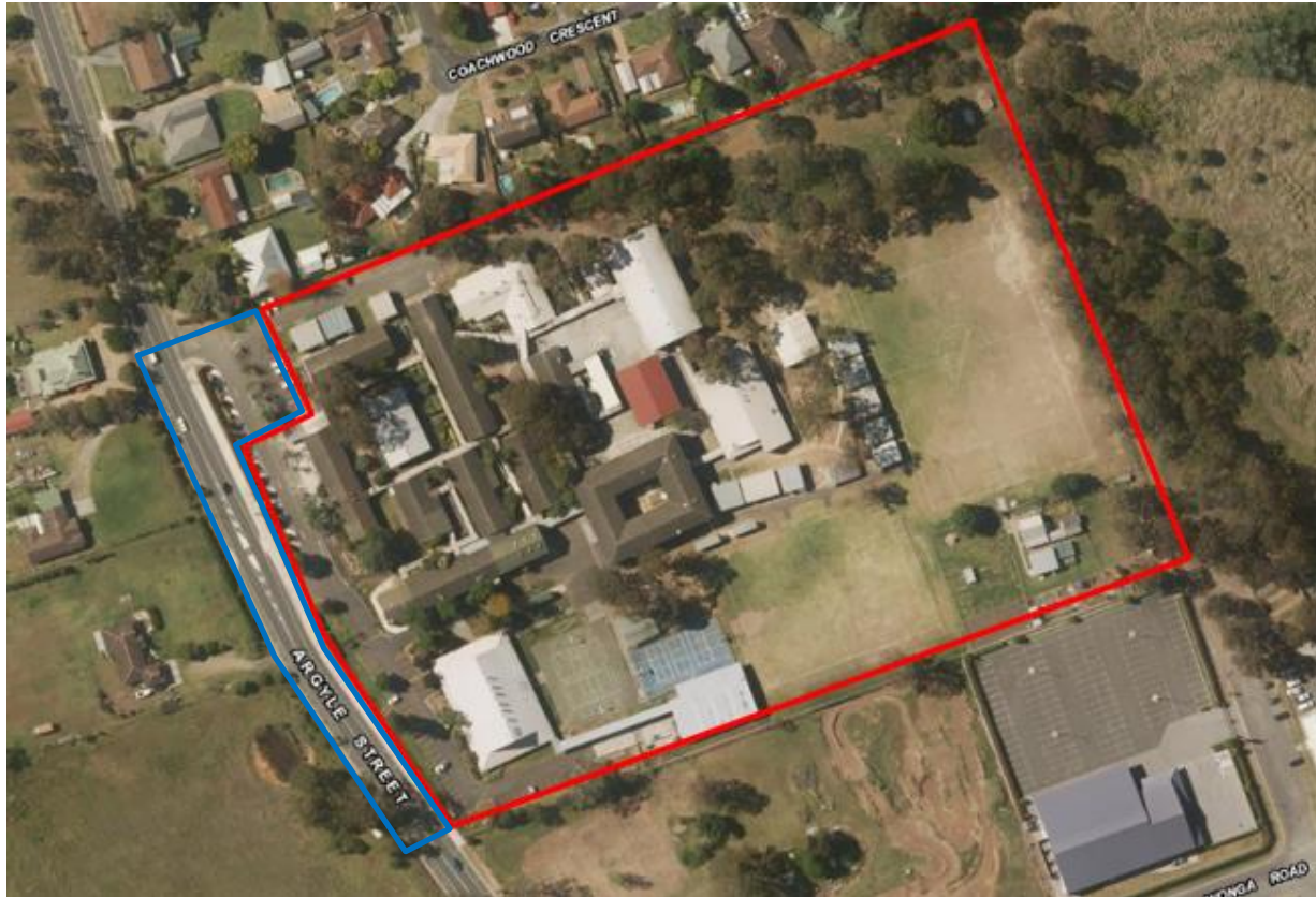
Figure 2 Aerial photograph showing general study site location and its frontage to Argyle Street. Study site approximately outlined in red. Works zone approximately outlined in blue. NSW Land and Property Information, Six Maps Viewer, accessed 19 th February 2019, https://maps.six.nsw.gov.au/
