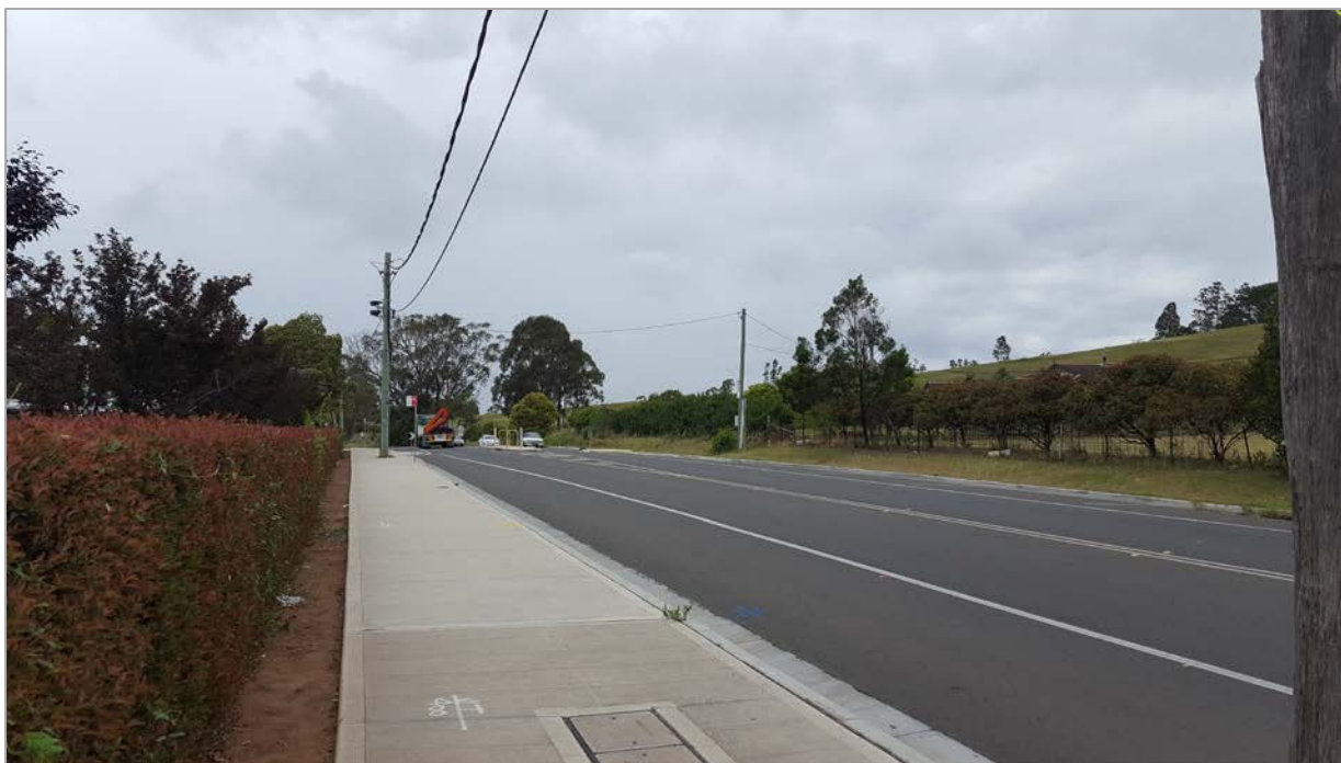
Photograph 5: Argyle Street providing primary access point on western boundary
