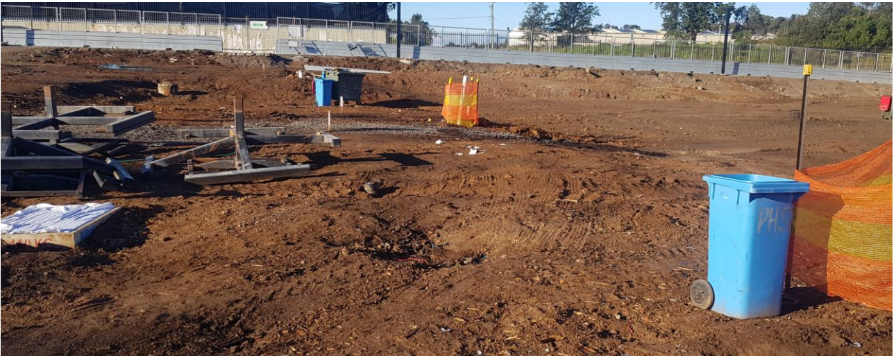
Photo 6: Clear, grub and investigations on Stage 3.
