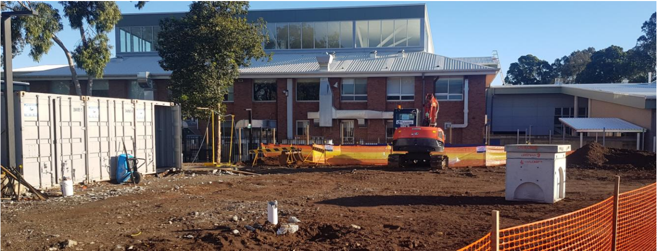
Photo 5: Stage 3 construction occurring adjacent operations of new school.
