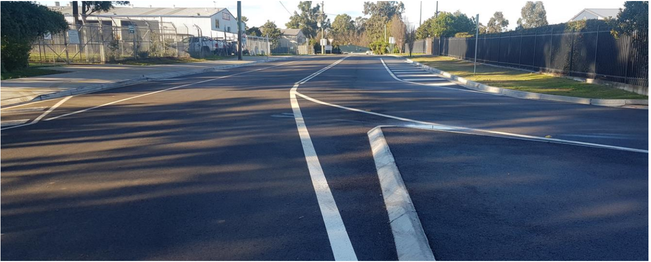
Photo 8: Wonga Road works complete.
