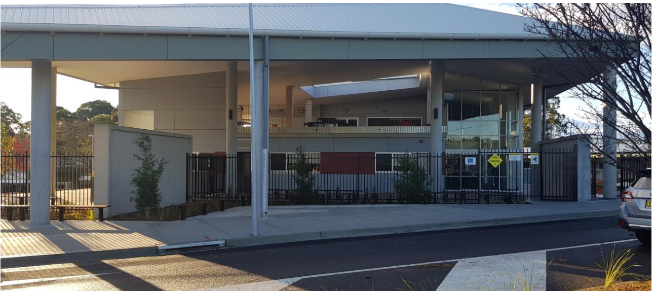
Photo 2: New school main entrance with kiss and drop and signage installed.
