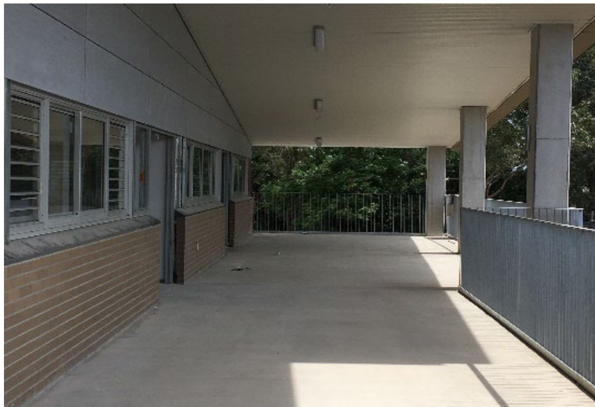
New Building E Covered Outdoor Learning Area
