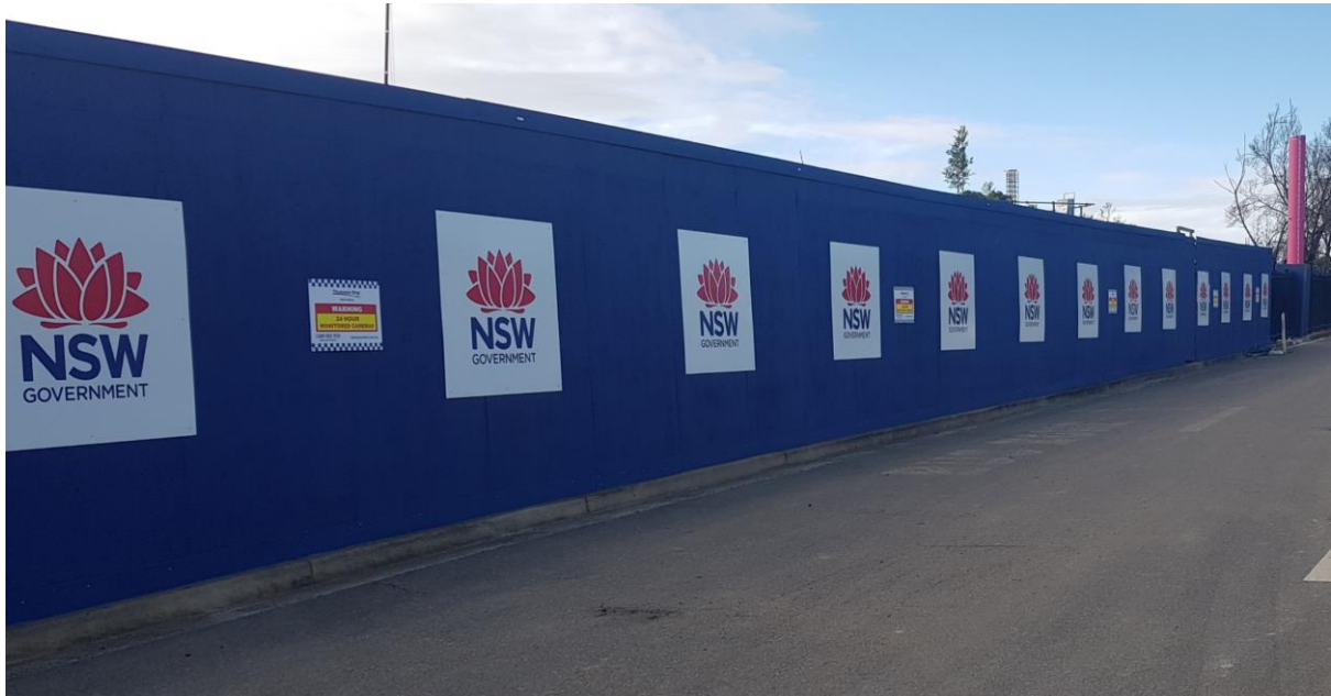
Photo 6: Site hoarding free of graffiti
