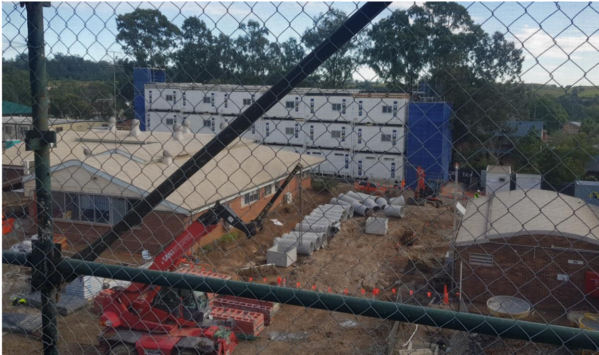
Photo 4: The three-story site sheds on the northern boundary adjacent to residential properties
