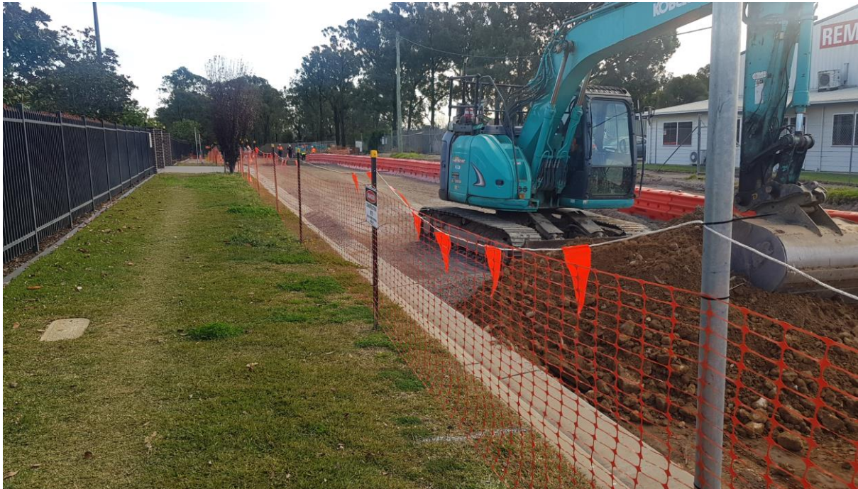
Photo 8: Wonga Road works with access to the left.
