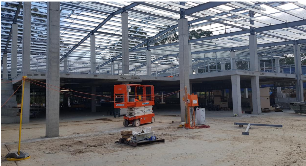
Photo 9: Main building structure erected with services being installed
