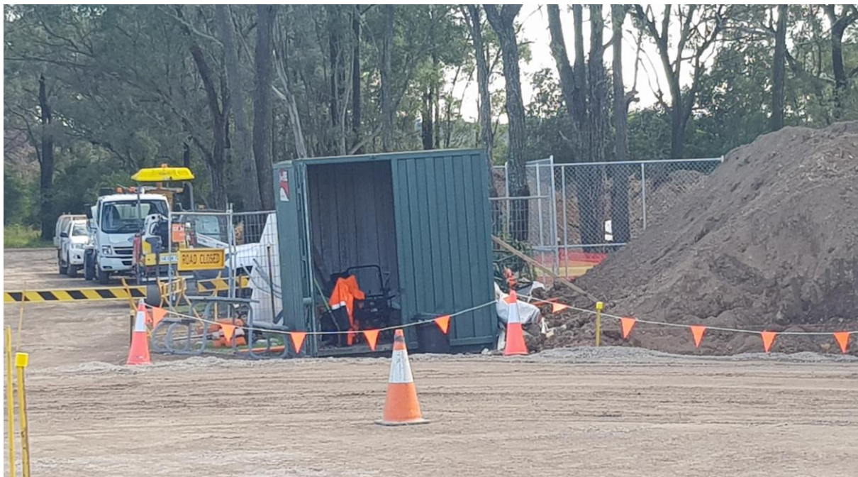
Photo 7: Wonga Road works – note stockpiles beyond the site boundary (fenced) in the background.
