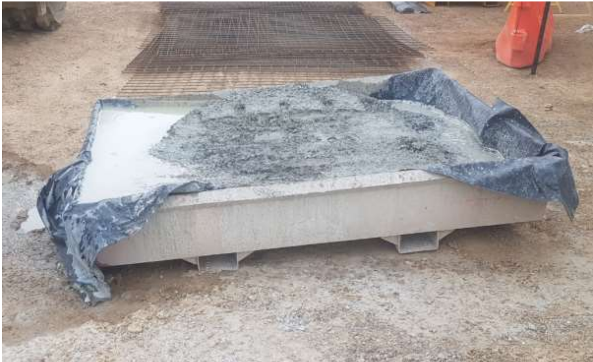
Photo 8: Concrete washout trays
