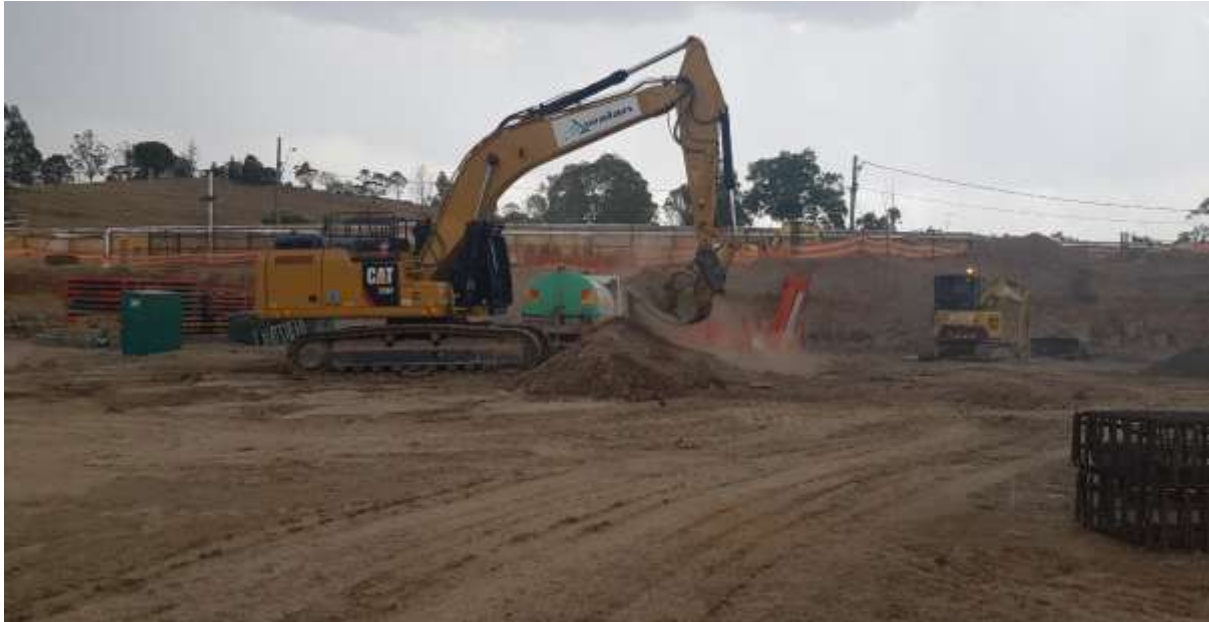
Photo 10: Material handling, note the dry conditions with watercart available
