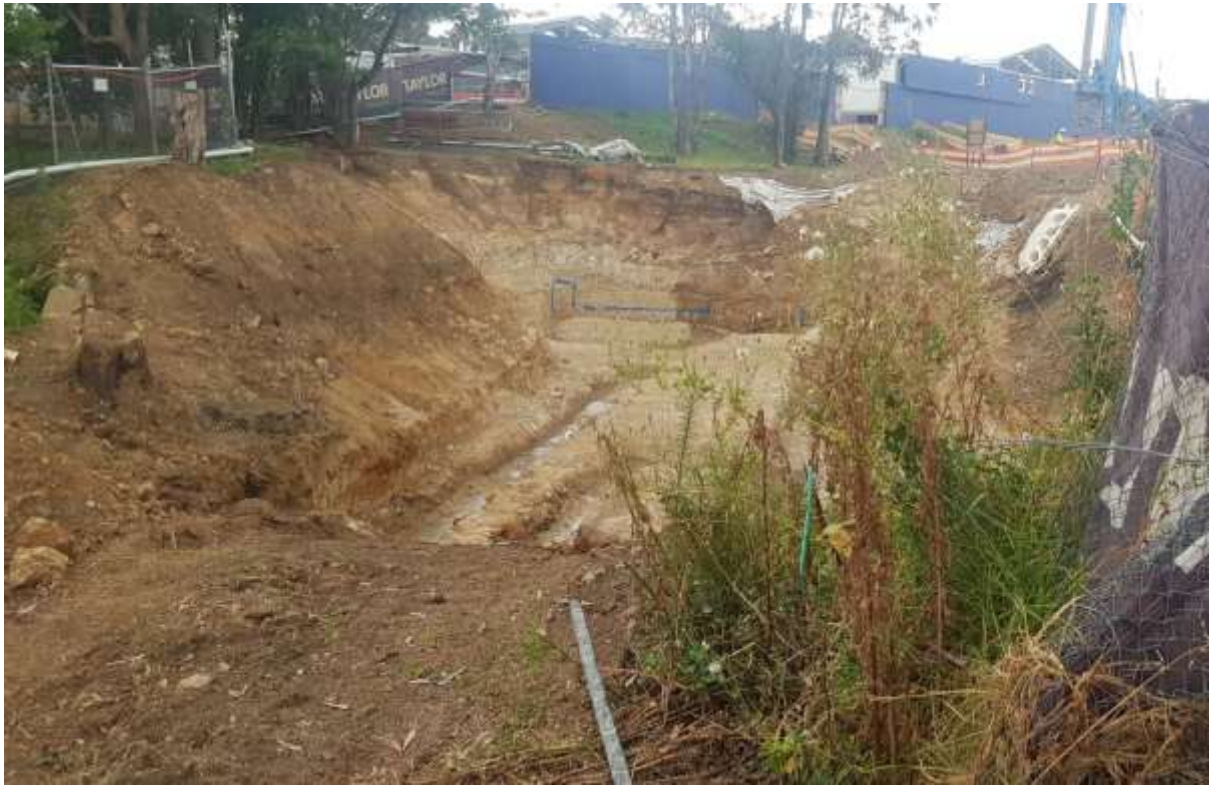
Photo 6: OSD installation works
