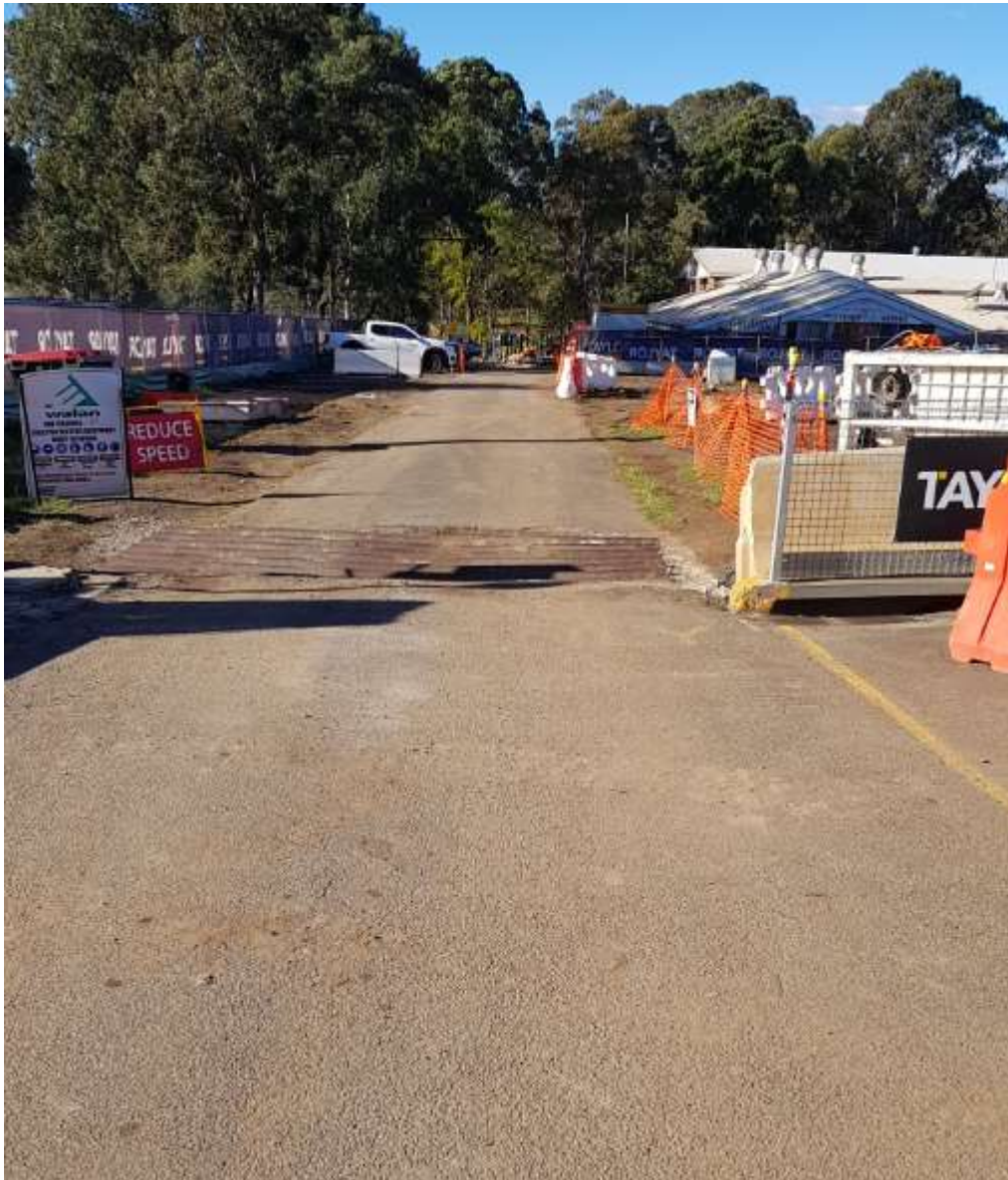
Photo 4: Stabilised site access
