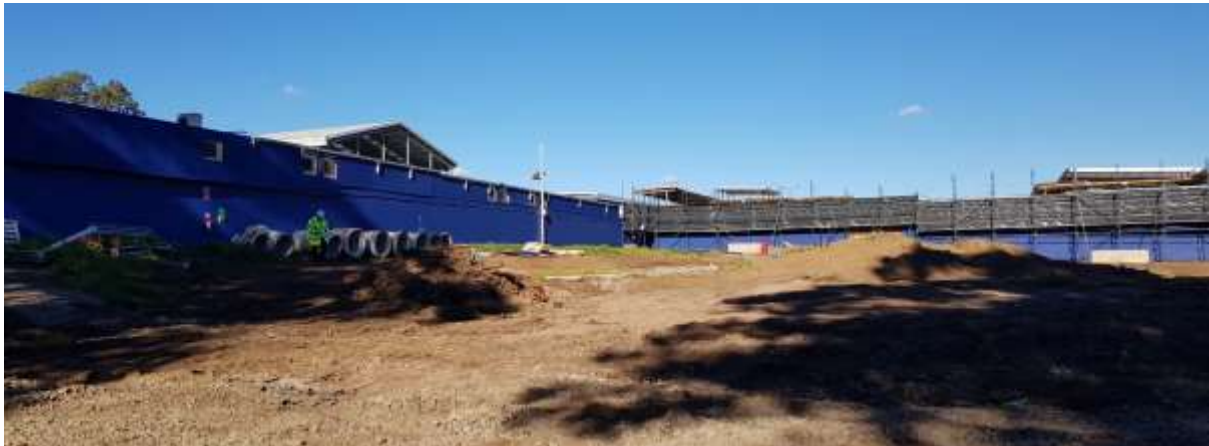
Photo 7: Noise barrier on temporary school boundary
