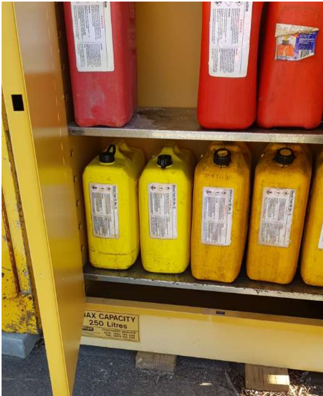
Photo 5: HAZCHEM storage with internal bunding
