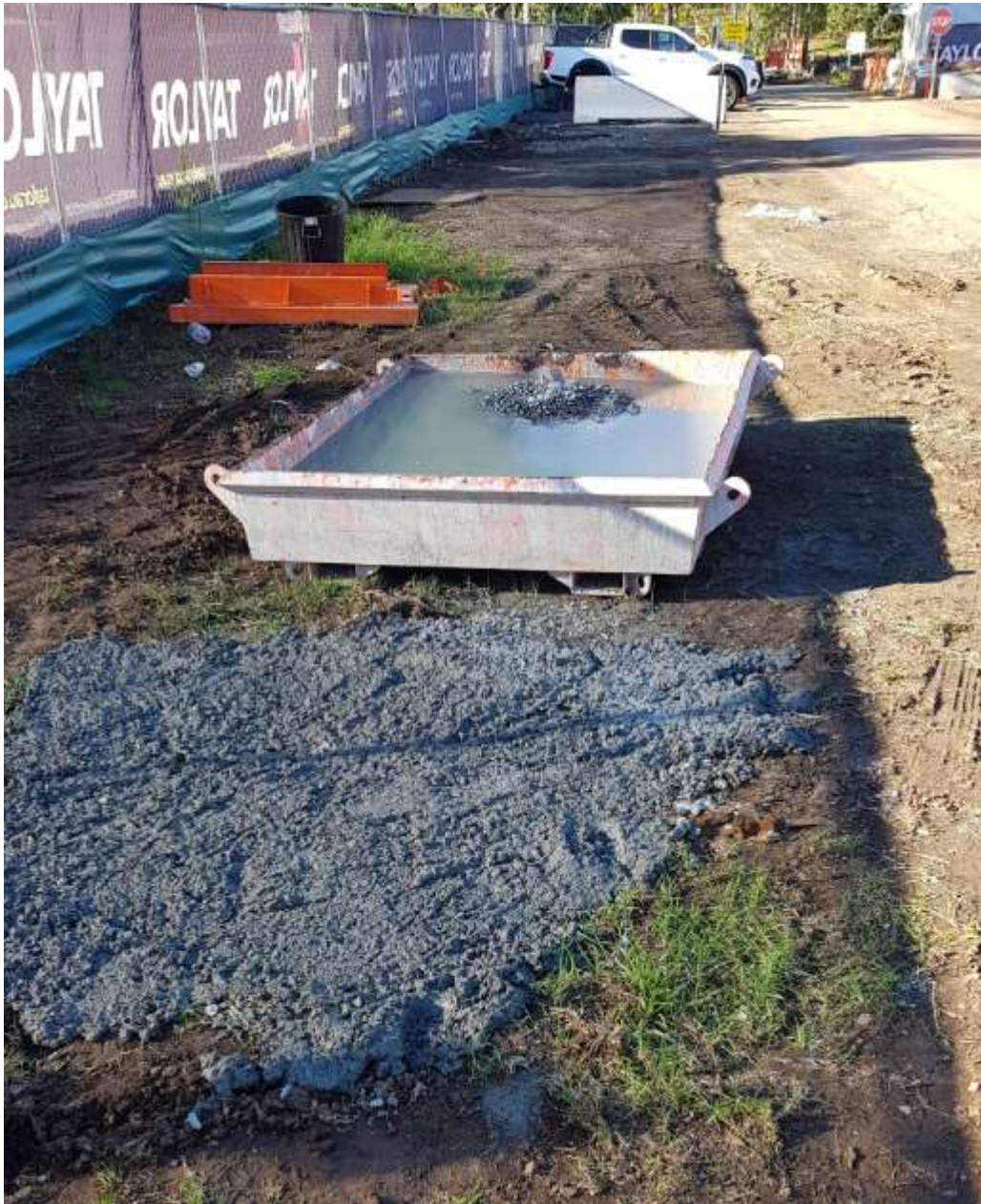
Photo 6: Concrete washout
