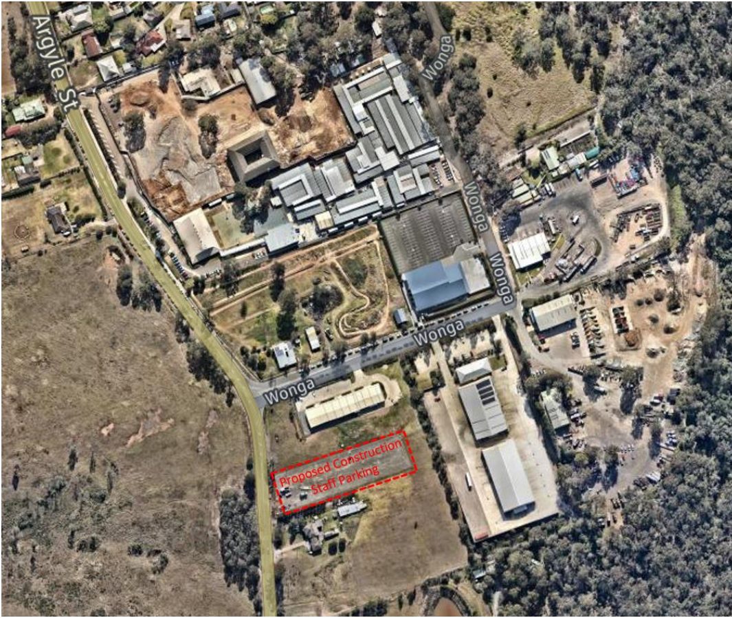
Figure 3-4: Proposed Construction Staff Parking
