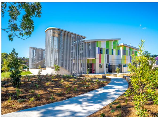
New Block L and landscaping works
