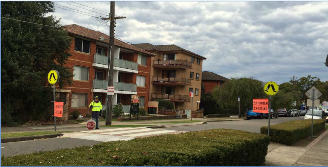
Figure 2-7: Children's crossing on Arcadia Street
