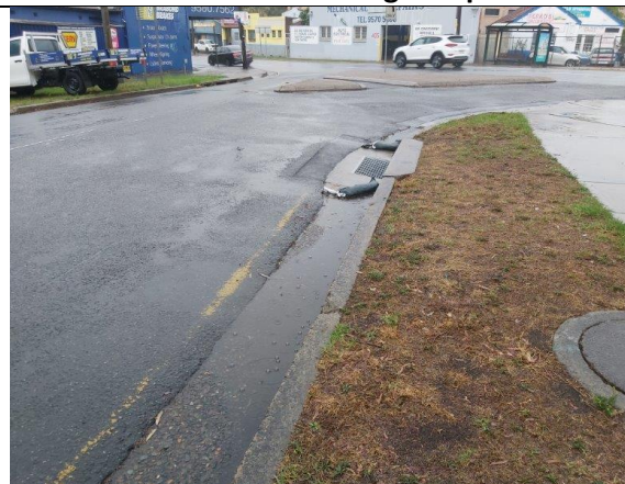
Wet weather controls during rain event
