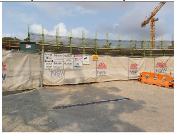
Stormwater inlet covered with geotextile fabric
