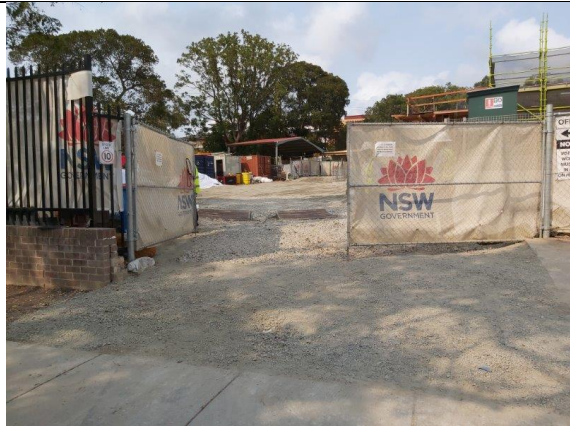
C23 – stabilised entry to site. ground, tracking of dirt (minimal)
