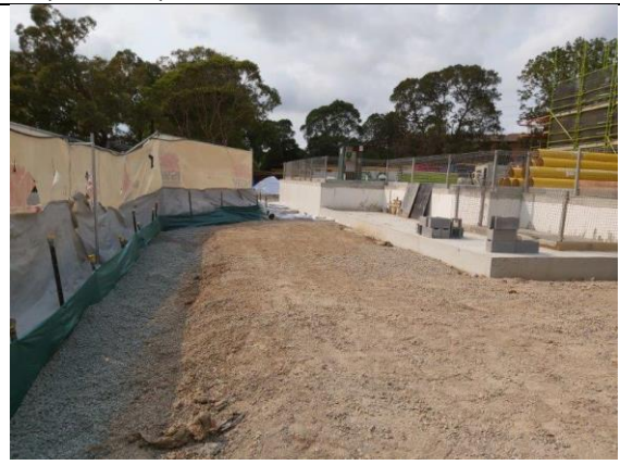
Erosion and sediment controls in place C25 and CEMP
