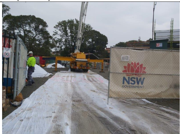
Geofabric laid out prior to wet weather work at entry to compound
