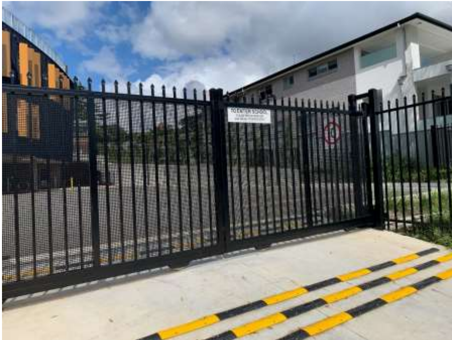
Figure 13 – Dedicated school carpark
