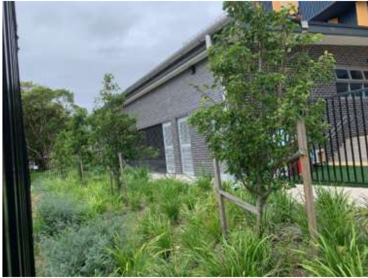
Figure 3 Final Landscaping Works
