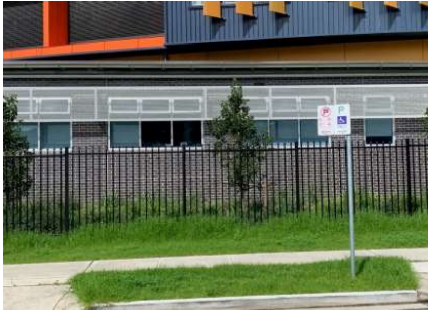
Figure 7 Parking restriction and disabled parking signage
