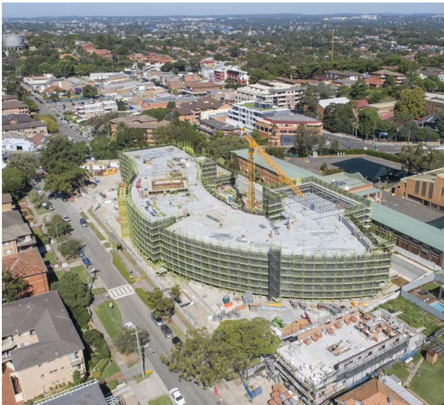
Peshurst Public School – structure of the new building structure completed April 2020
