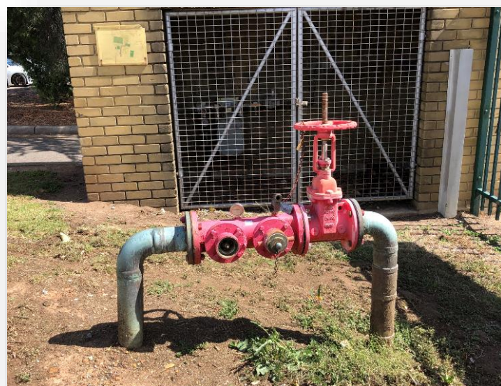
Figure 12: Fire Brigade Booster Assembly
