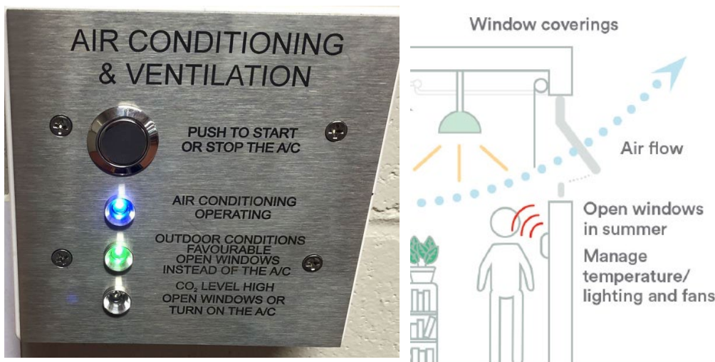
Figure 5 Indicative light system proposed and natural ventilation illustration (SI NSW, GA NSW)
