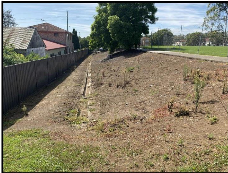
Figure 24: [Image position 1] The northern edge of the sports field with exposed fill consisting of broken shale from bedrock mixed with fill material.
