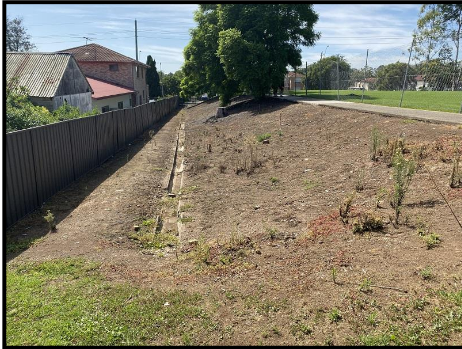
Figure 25: [Image position 1] The northern edge of the sports field with exposed fill consisting of broken shale from bedrock mixed with fill material.
