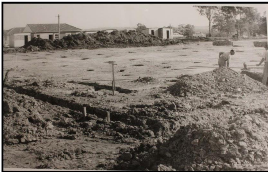
Figure 19: Ground prepared for construction platforms. Courtesy NSW State Records. 1964-65 Pendle Hill High School Photos NRS-15051-1-26-[1468] 267 - OPA
