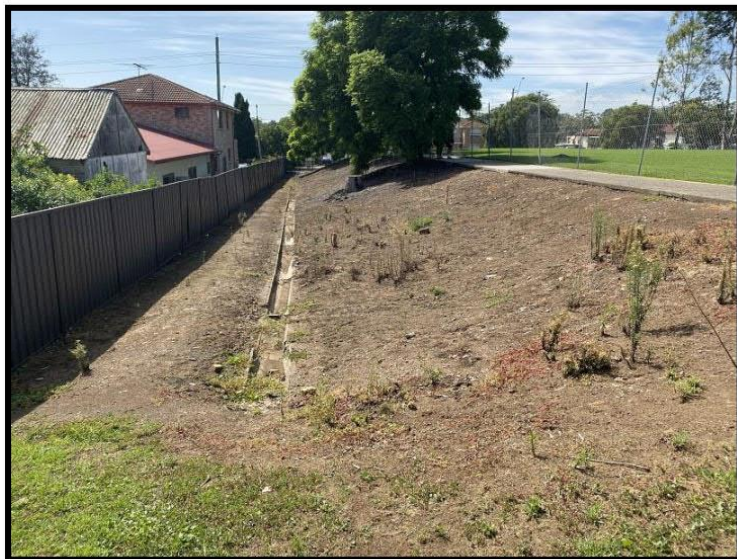
Figure 23: [Image position 1] The northern edge of the sports field with exposed fill consisting of broken shale from bedrock mixed with fill material.
