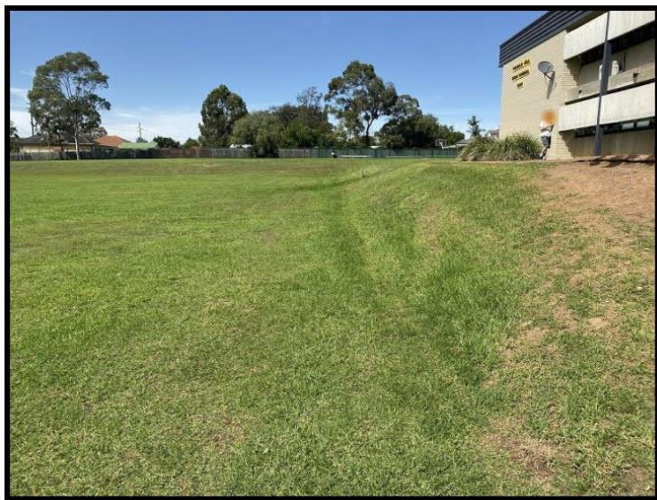
Figure 24: [Image position 2] Levelled sports field and batter leading to the building platform.
