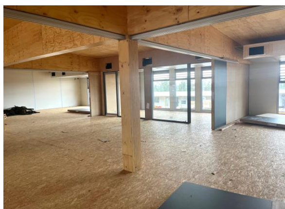
Interior view of classroom in progress
