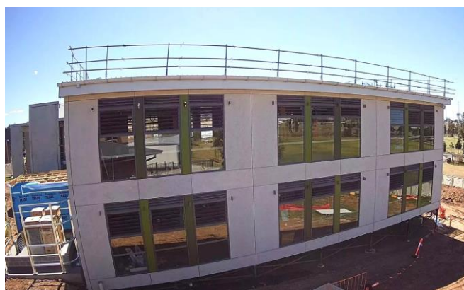
Exterior view of classroom building O in progress
