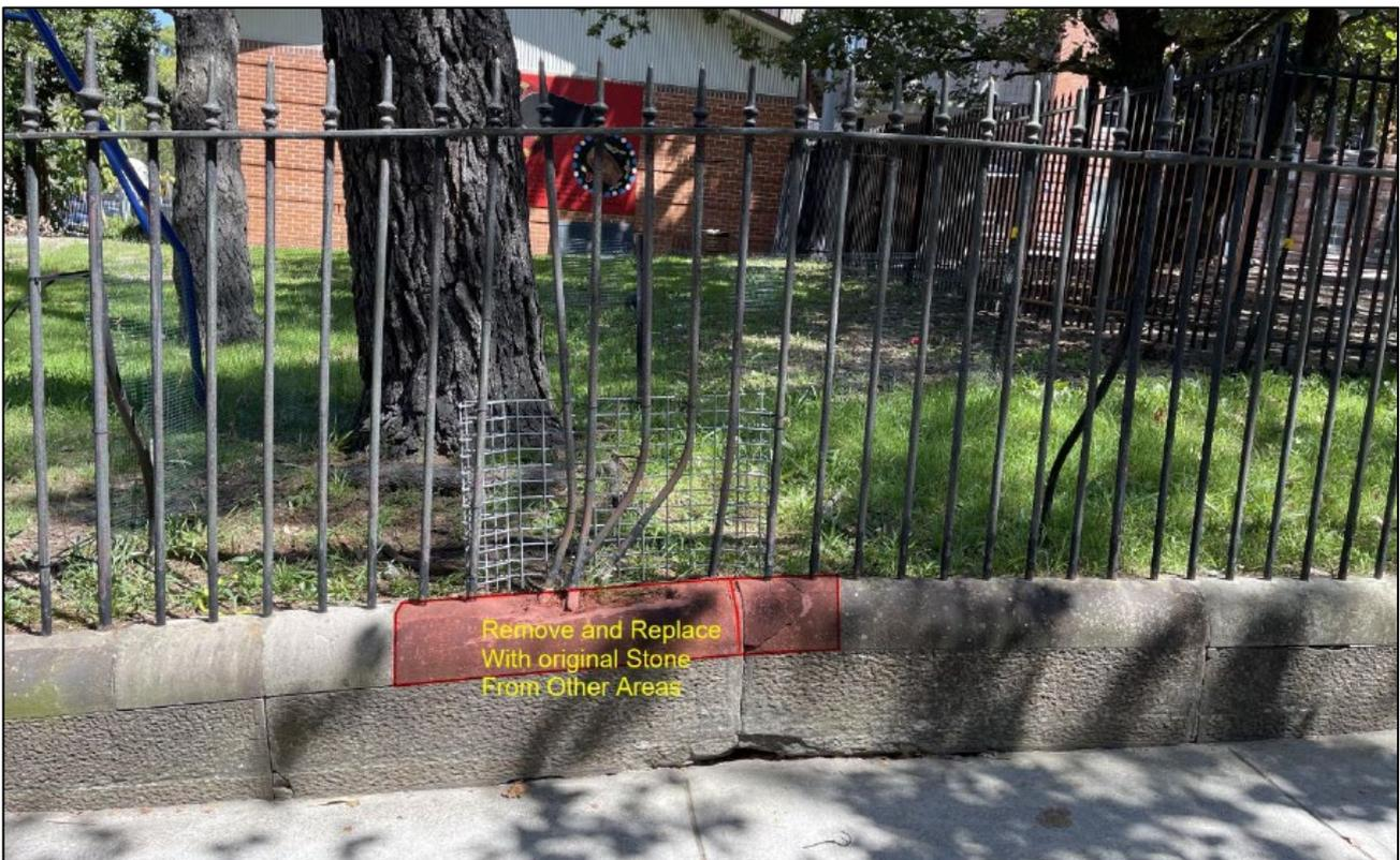
Figure 7 | Extent of sandstone repair works (Source: Modification 3, 2023)
