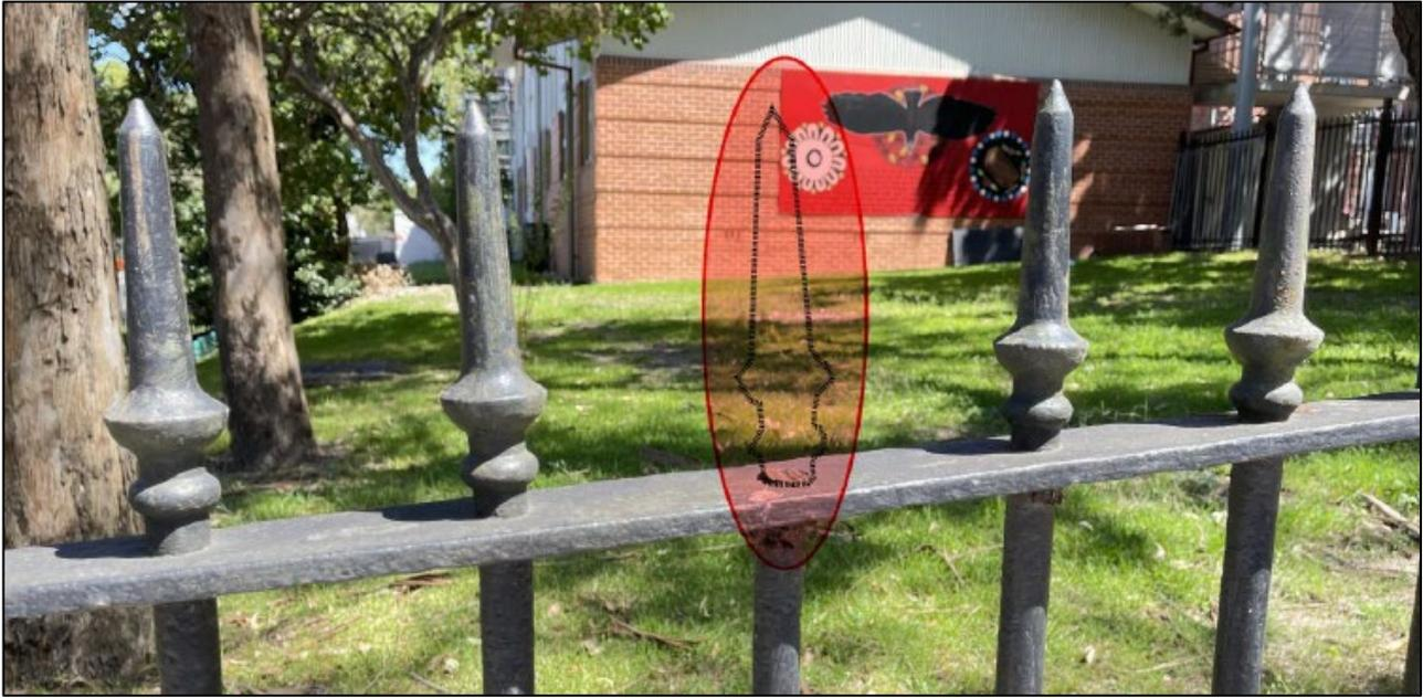
Figure 6 | Missing finial to be replaced (Source: Modification 3, 2023)
